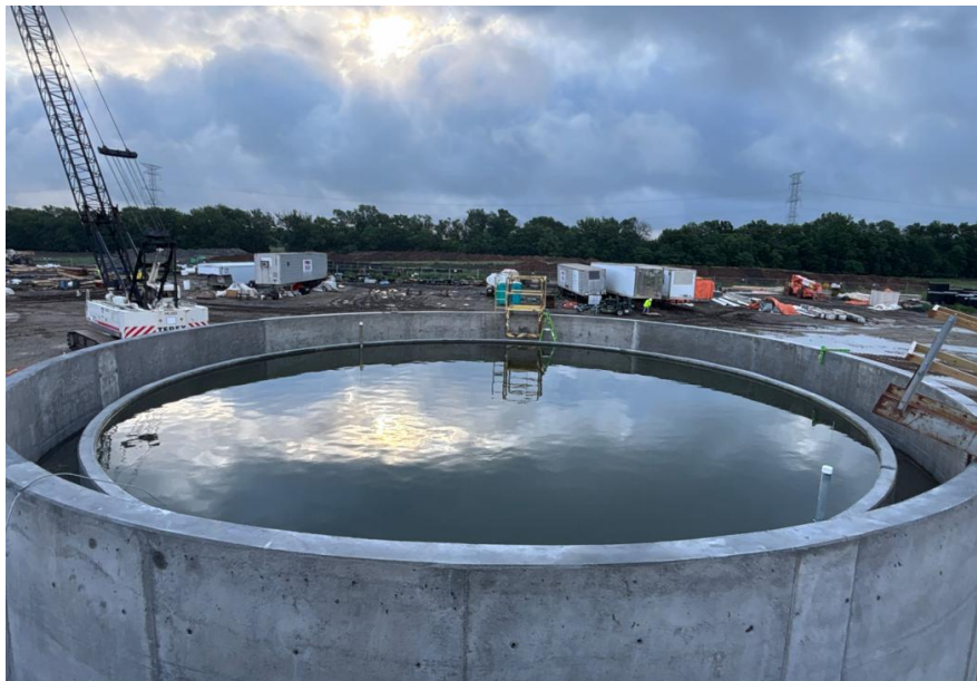
Clarifier #3 – Water Tightness Testing
