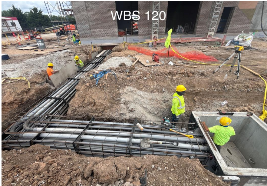
Electrical Duct Bank Installation
