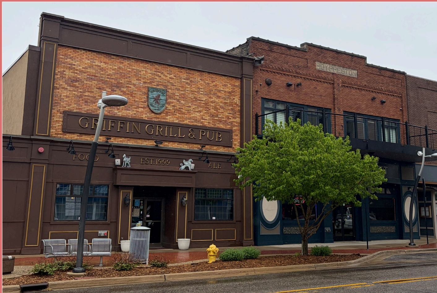
Many of the commercial buildings in the Central Business District have masonry facades and masonry detailing. Photo by Loggia Preservation, 2026
