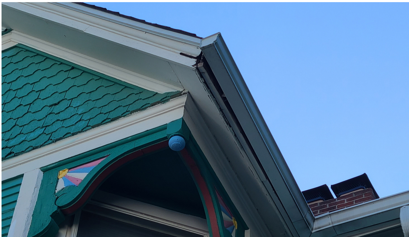
West side (facing neighbor)
