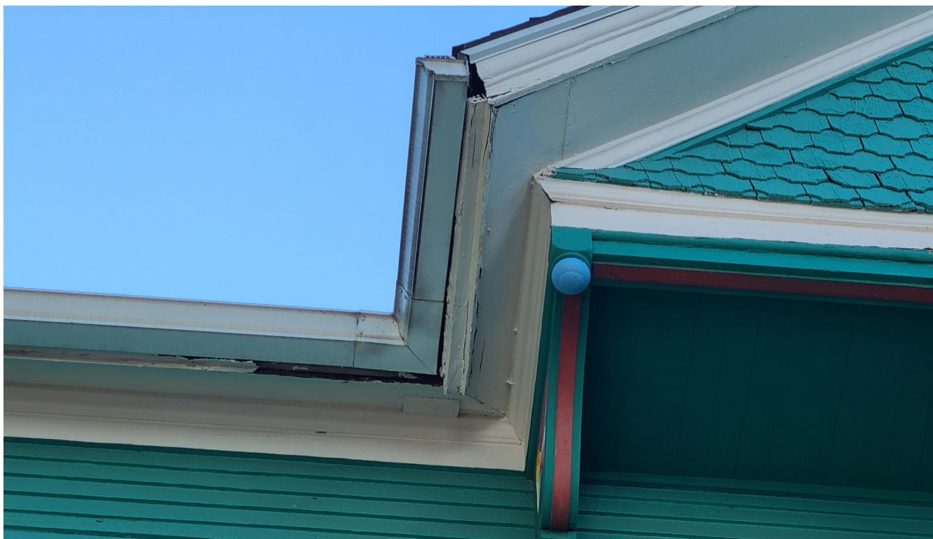
West side (facing neighbor)
