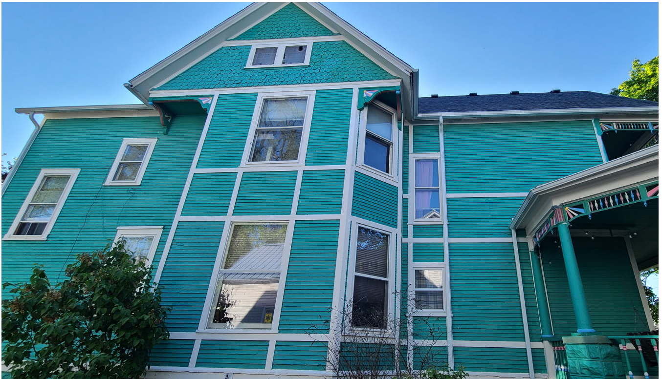
West side (facing neighbor)
