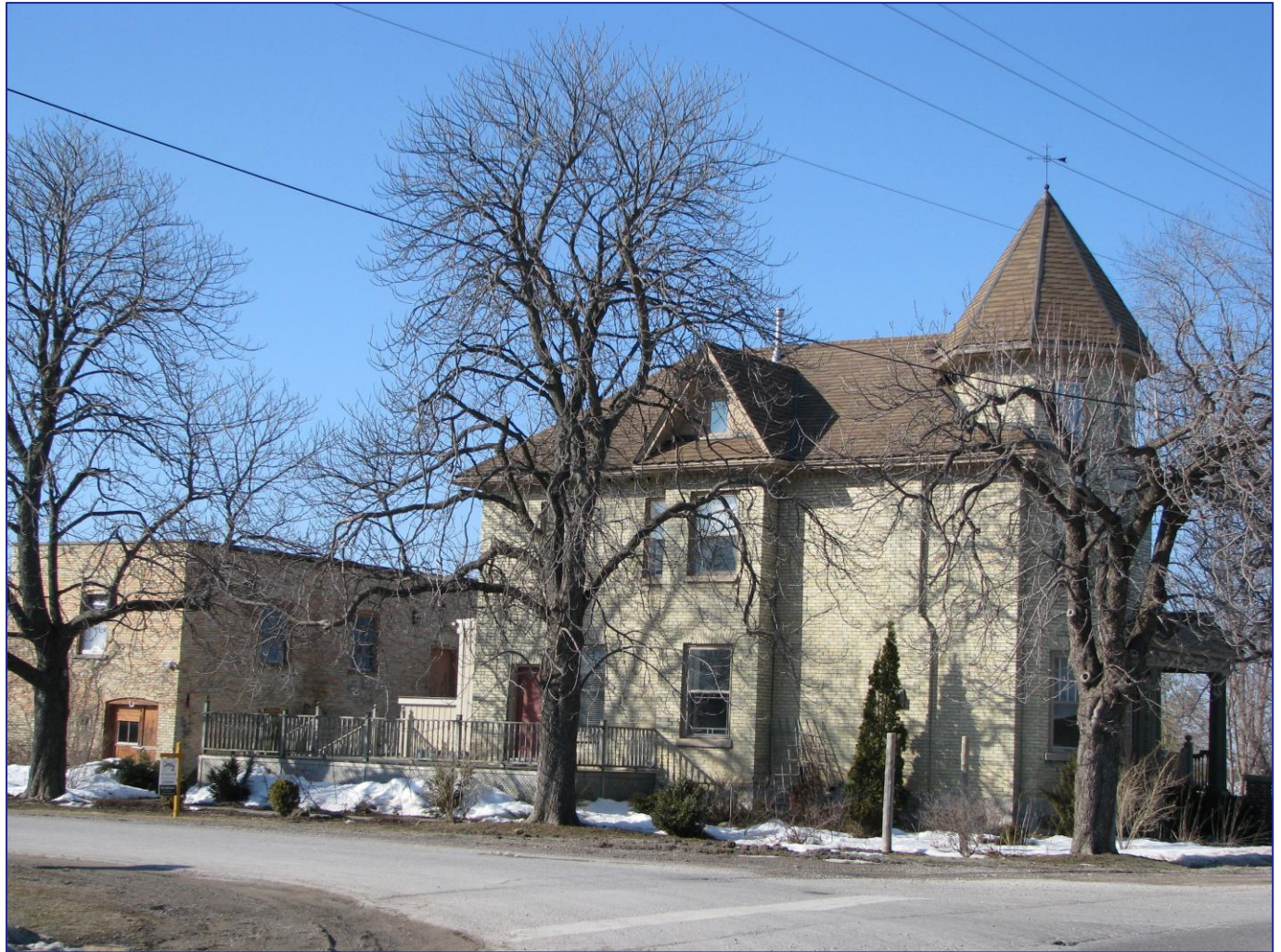
Municipal file photo of property known as The Organ Factory. The flat-roofed building is a remnant of the founding of St. Joseph by Narcisse Cantin, who dreamed of building a canal to connect Lake Huron to major shipping routes.
