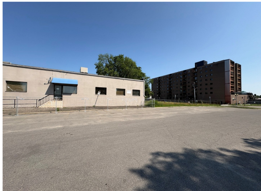
5 Home Street – Looking North towards 3 Apple Street.
