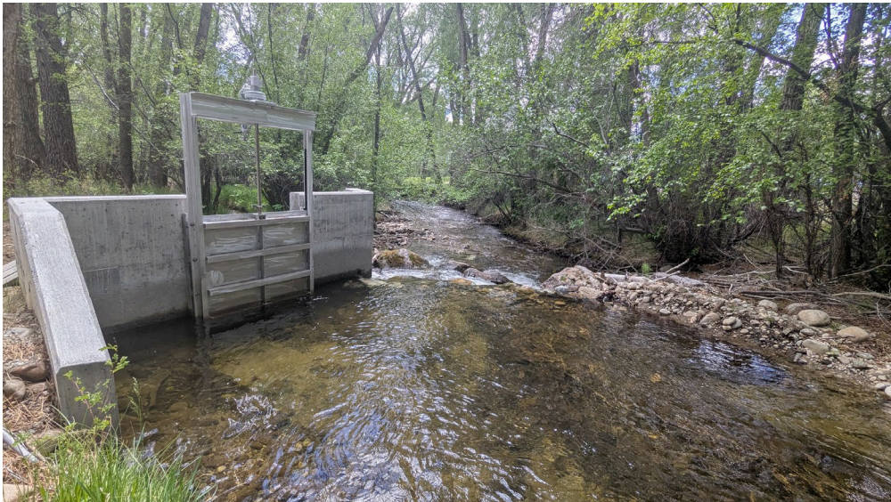
Gorrel Head Gate North Cottonwood Creek
