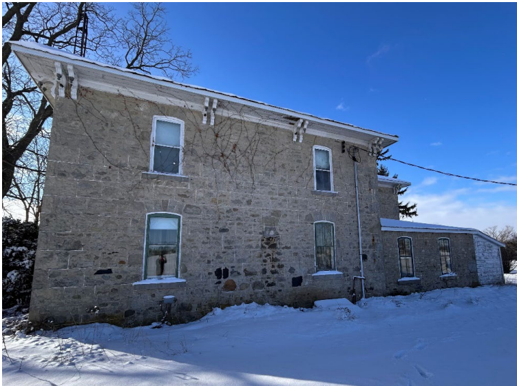
Figure 82 side façade (east elevation)side façade (east elevation)
