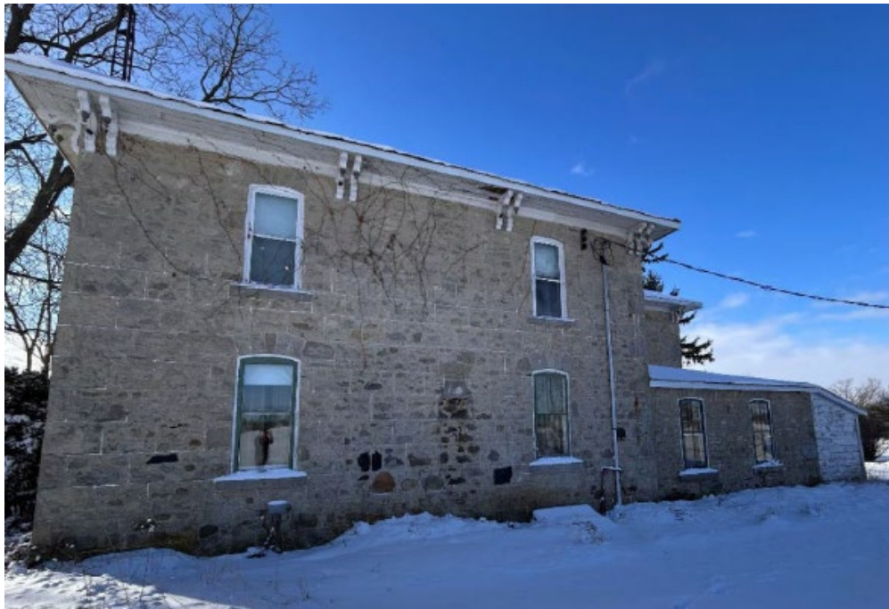
PHOTO 4: 2-Storey Dwelling Side (East) Elevation (MHBC 2025)
