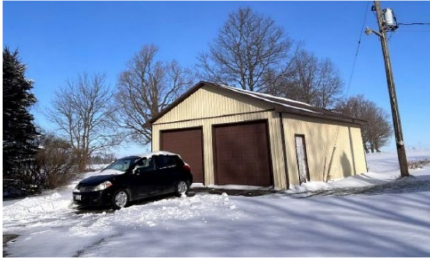
PHOTO 7: Metal Clad Frame Garage (MHBC 2025)
