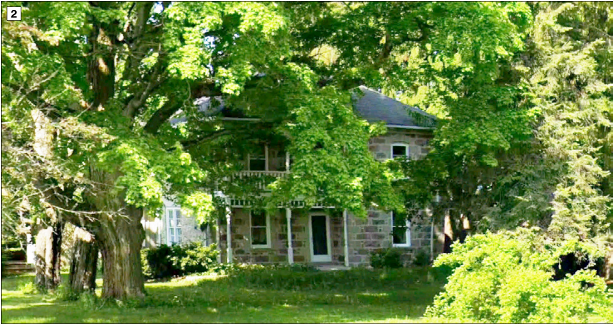
1. View of stone Italianate dwelling located at 7122 Wellington Road 16;
