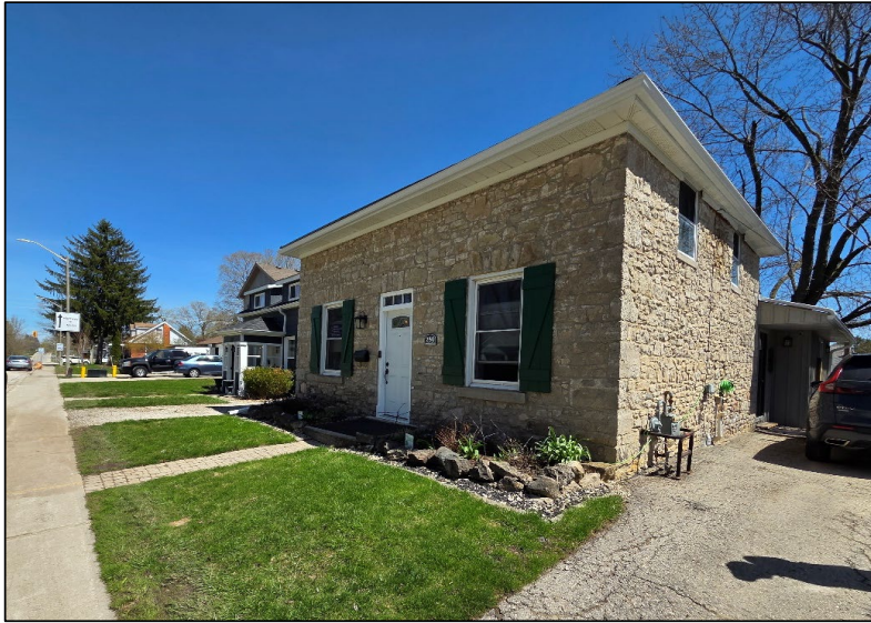
Photo 3: Northwest corner of the dwelling
