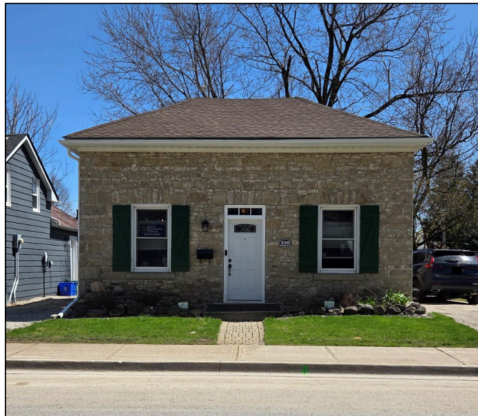
Photos 1 & 2: Front façade facing north (Spring 2026)
