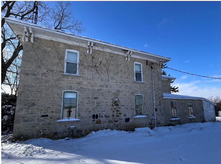
Figure 82 side façade (east elevation)side façade (east elevation)
