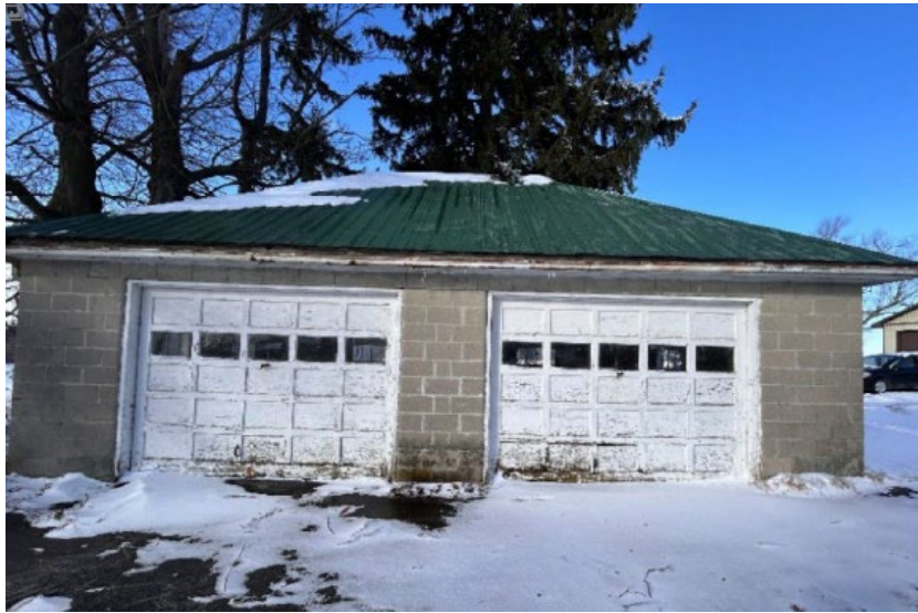
PHOTO 8: Concrete Block Garage (MHBC 2025)
