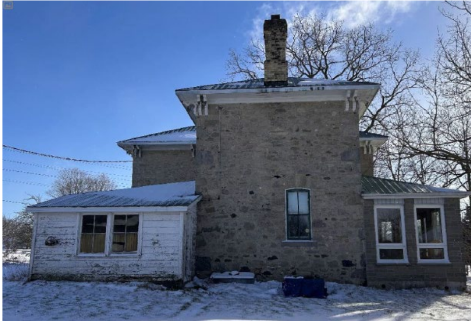
PHOTO 5: 2-Storey Dwelling Rear (North) Elevation (MHBC 2025)
