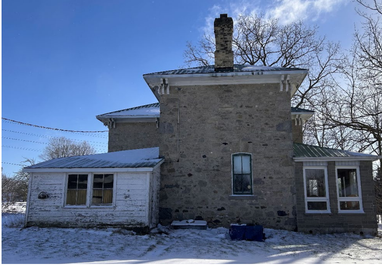
Figure 10.9 rear façade (north elevation) rear façade (north elevation)
