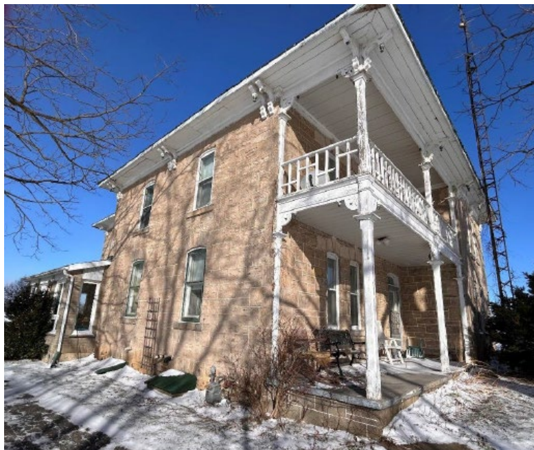
PHOTO 6: 2-Storey Dwelling Side (West) Elevation (MHBC 2025)
