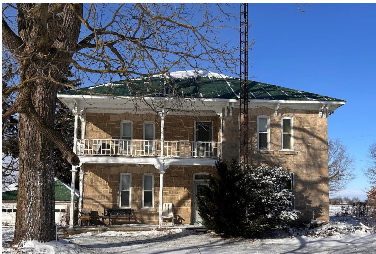
Figure 66: Front façade (south elevation) front façade (south elevation)
