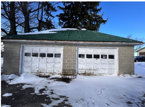
Figure 12: Concrete block garageConcrete block garage
