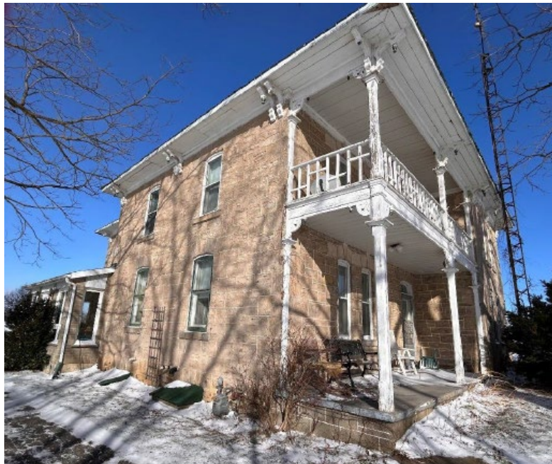
PHOTO 6: 2-Storey Dwelling Side (West) Elevation (MHBC 2025)
