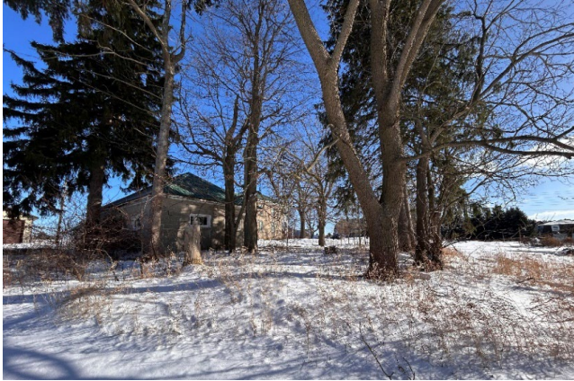
Figure 15-1 Cluster of trees behind the block garage
