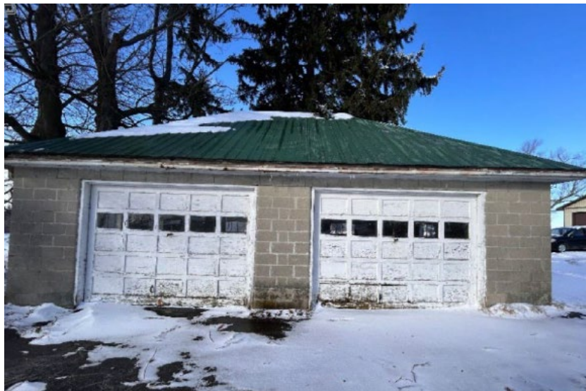
PHOTO 8: Concrete Block Garage (MHBC 2025)
