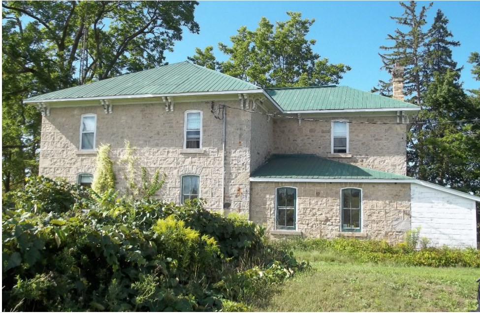
PHOTO 3: 2-Storey Dwelling East Elevation (Township 2017)
