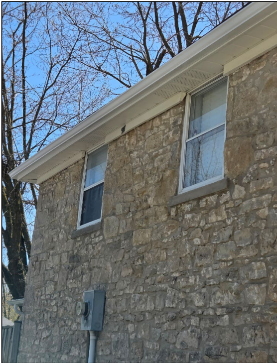
Photo 4: East facing façade
