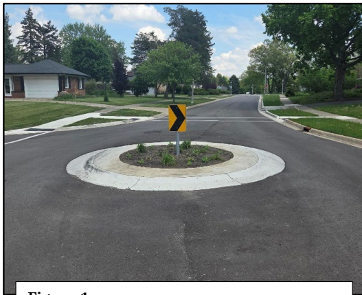
Figure 1: Traffic circles provide obstructions which require drivers to slow down to navigate around them. They can be placed in most intersections without changing the geometry of the curbline. Similar measures can be found in the Bailey Neighborhood.
