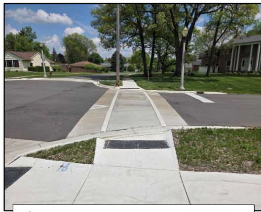
Figure 2: Raised crosswalks provide elevated surfaces which require drivers to slow down to navigate over them. Special emphasis pavement markings are typically used in conjunction with the structure to draw attention to the presence of the device.
