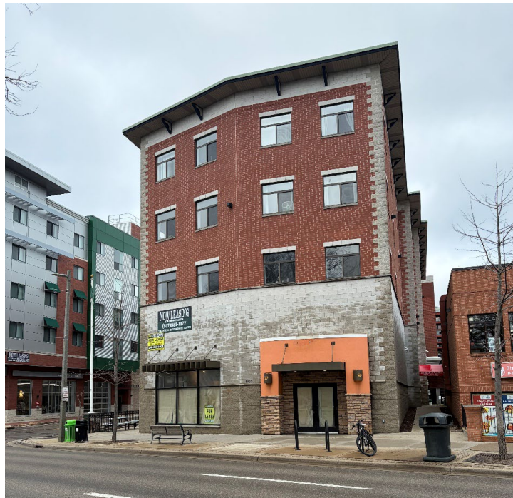
Site photo taken April 3, 2026, from south side of Grand River Ave.
