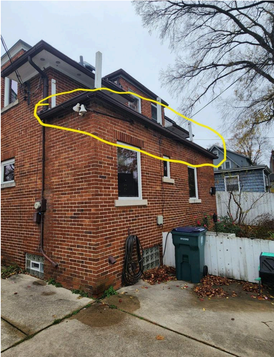
Where the gutters are being replaced - KSTYLE BLACK 5" ALUMINUM GUTTERS ~20ft
