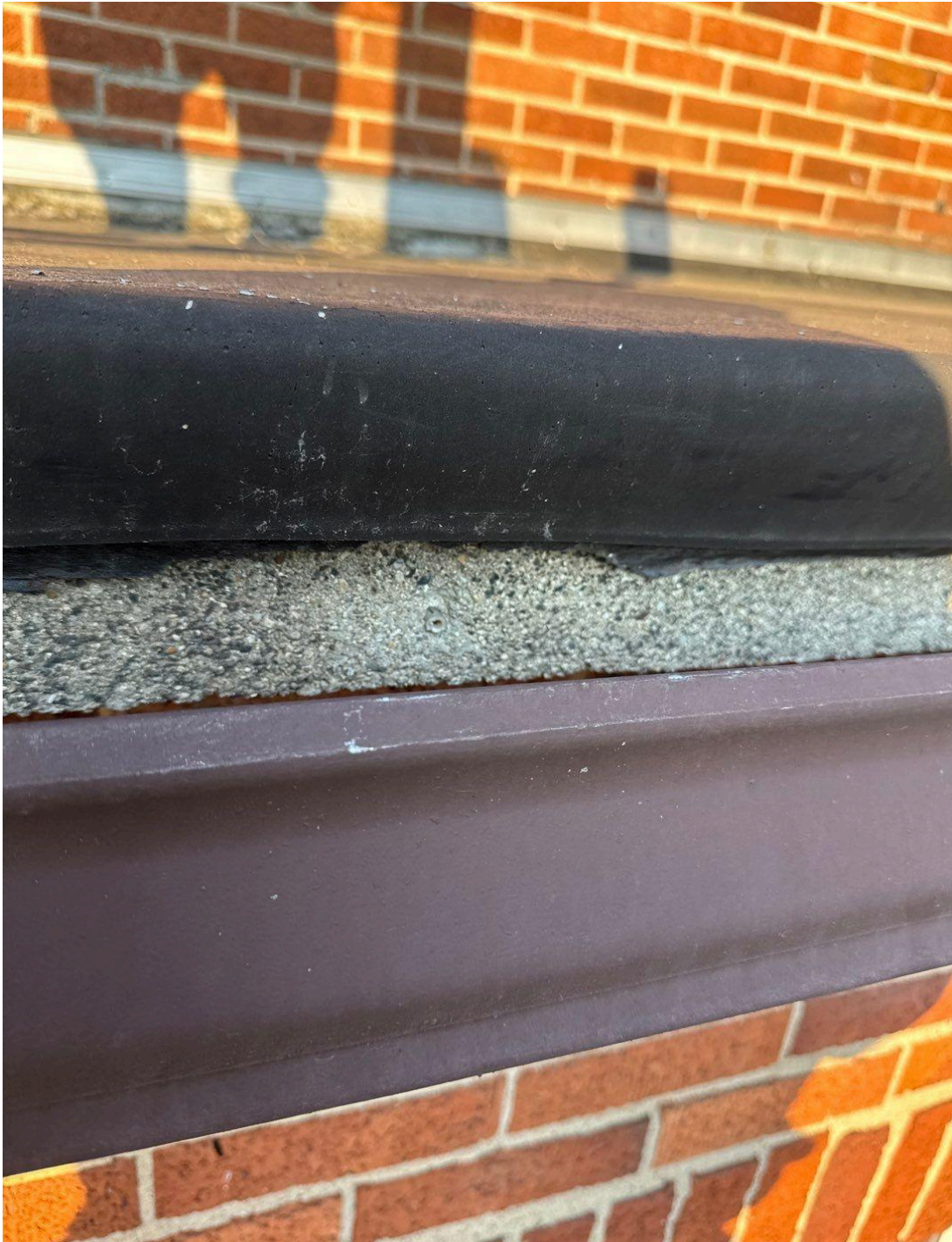
Where the 2x6 is going
