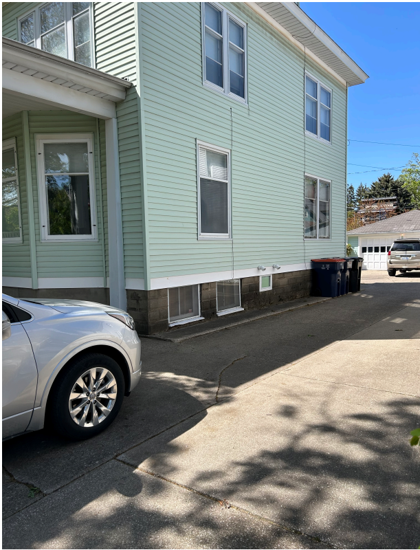
Right side of house, windows 1 and 2.
