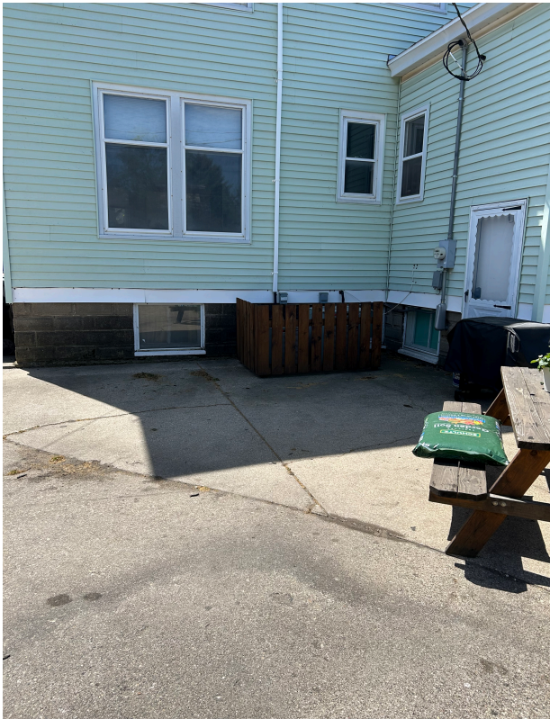
Back of house, Windows 3-5. Window 4 is hidden by the air conditioner.
