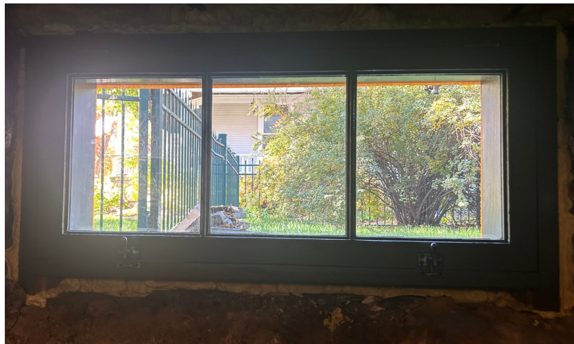
Restored window in place
