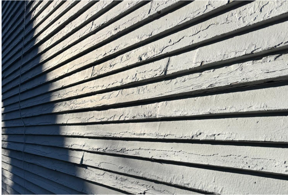
Figure 8: Existing cedar clapboard siding at 276 Pine Ave, showing the 3½-inch beveled profile and current condition. The siding requires sanding and repainting; the cedar substrate and profile are sound and will be preserved and matched on the addition.
