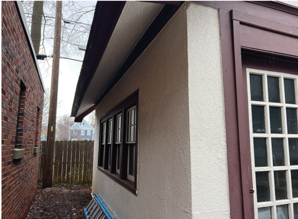
Existing Garage: West View
