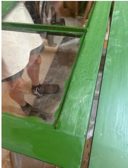
Restored window frames after priming
