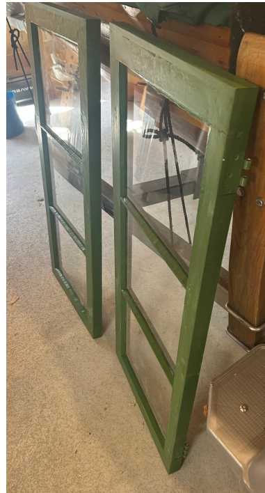
Restored window frames after priming
