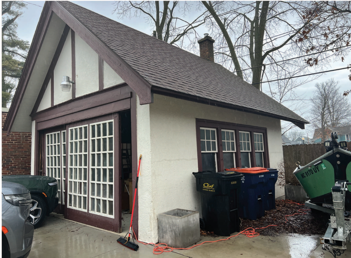
Existing Garage: South and East View
