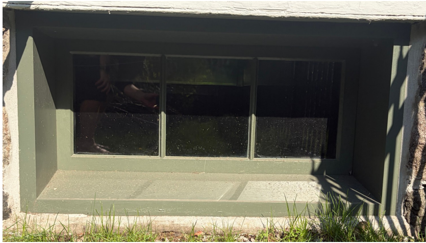
Restored window in place
