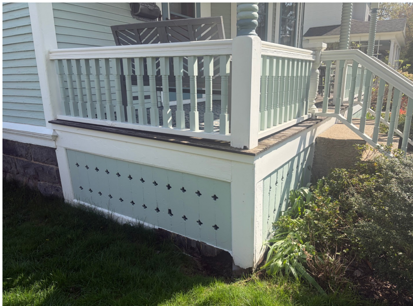
Porch viewed from the South West
