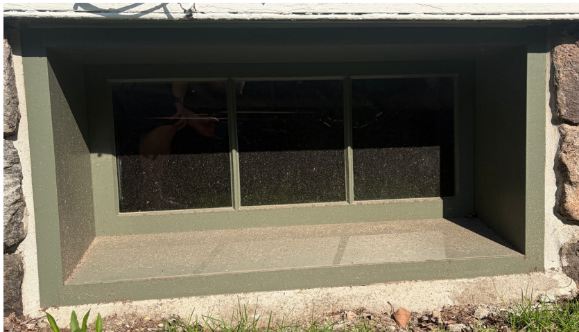
Restored window in place
