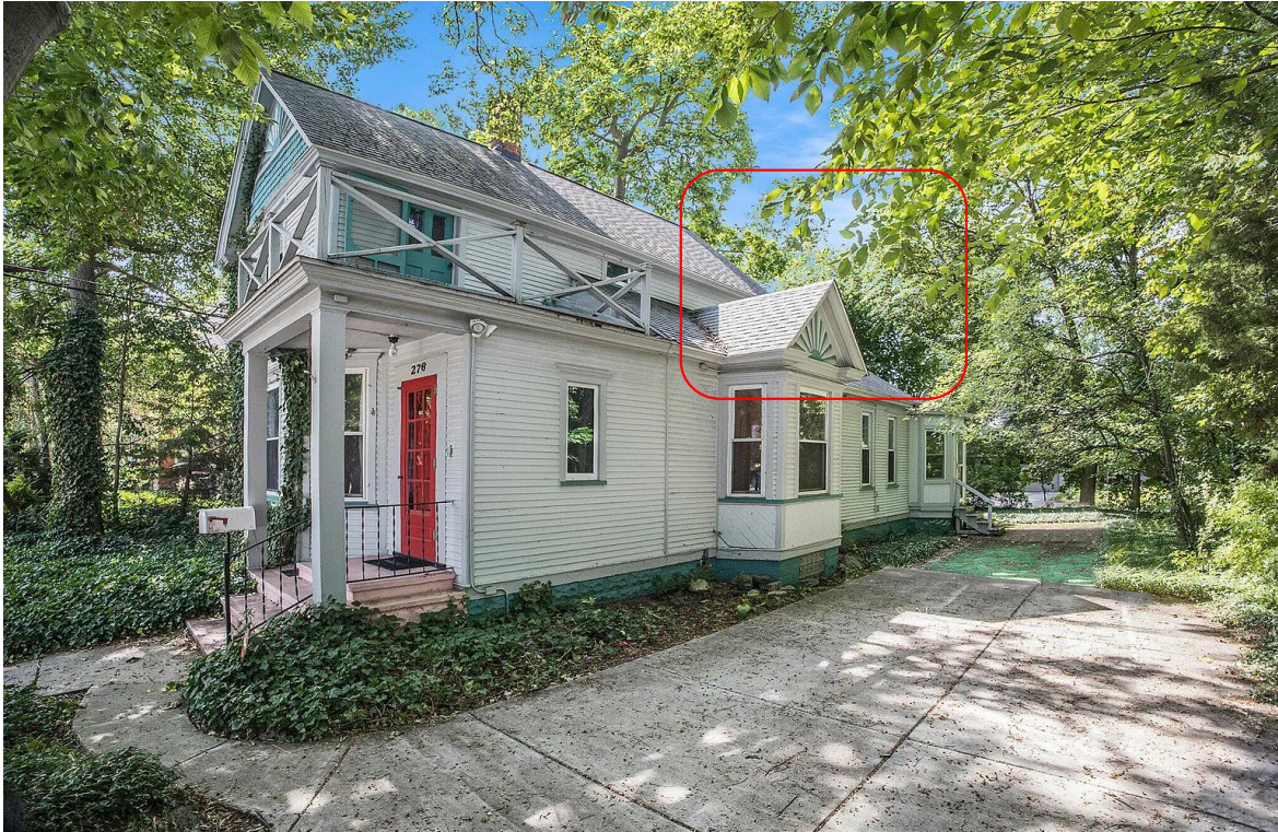
Figure 1: Existing front view of 276 Pine Ave. Red outline indicates the lower rear roofline of the current attic, the area proposed for the addition. Mature trees screen the rear of the property from the street.
