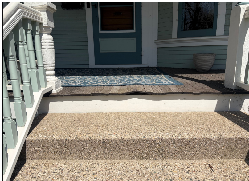
Details: Front Stairway – Current Condition
