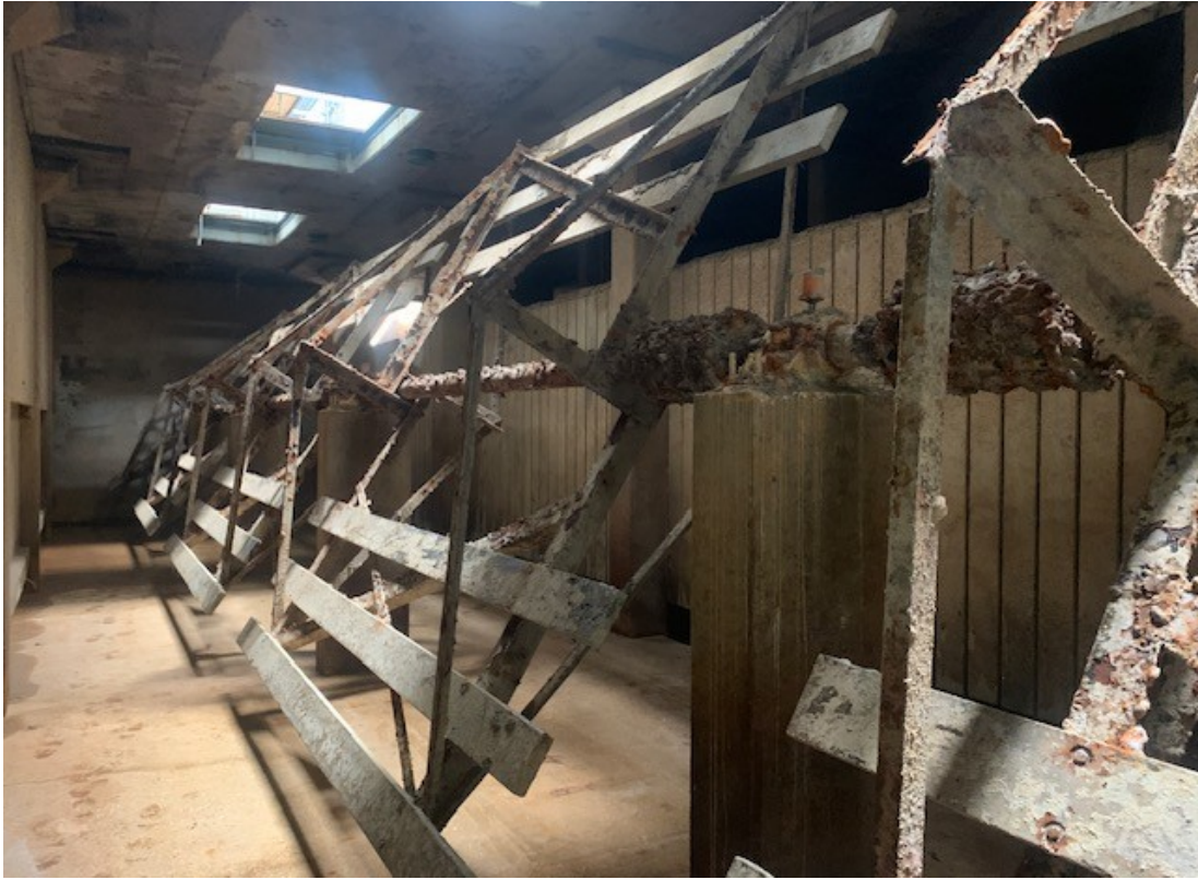
Original redwood paddle shafts, bearing housings, and support structure
