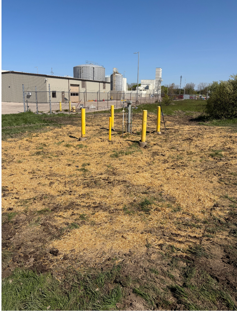
Excavation and bollards back in place, project complete
