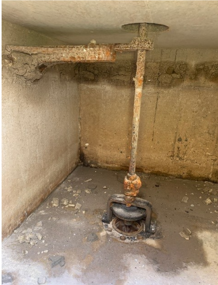
One of 7 original mud drain valves
