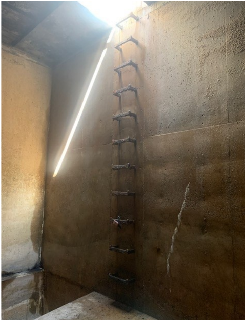
Original 1970s basin entrance ladder
