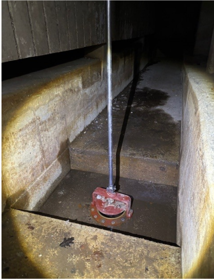
One of 7 newly replaced mud drain valves
