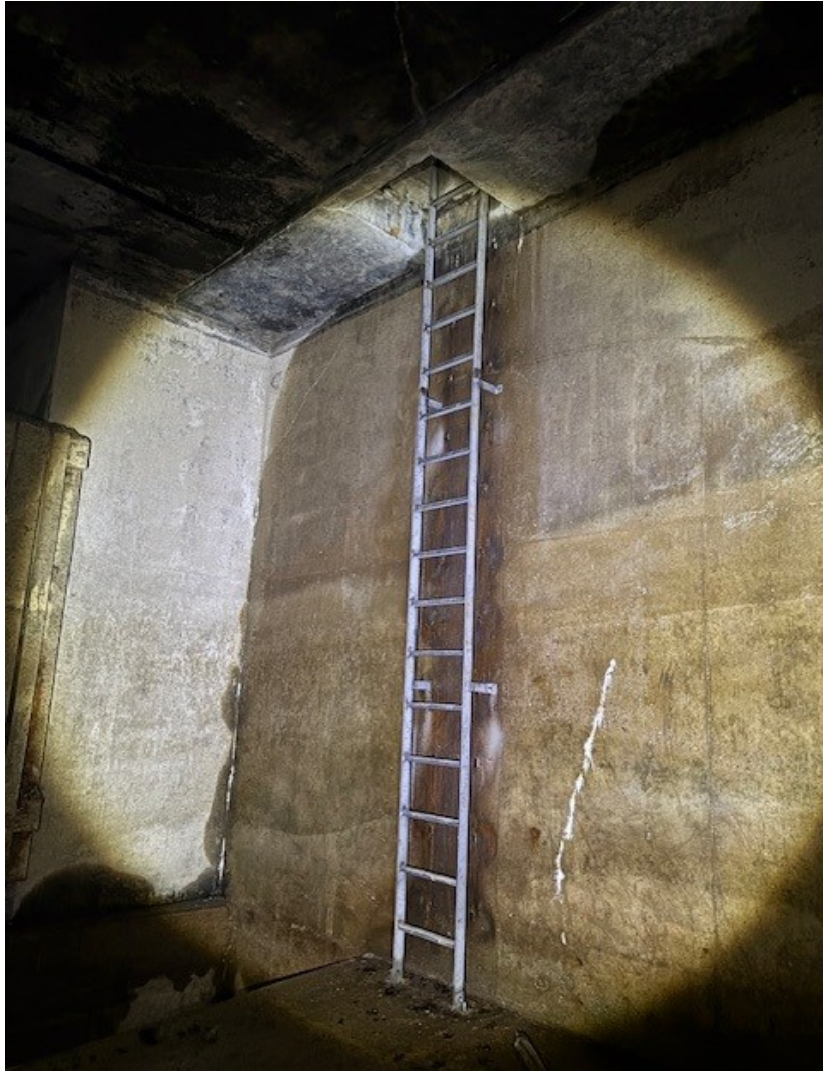
New stainless steel basin entrance ladder
