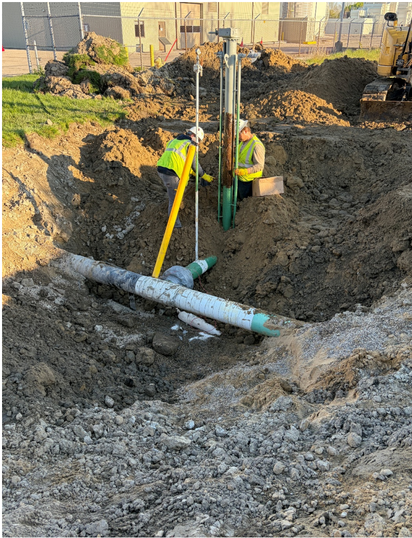
Underground pipe wrap and sealant
