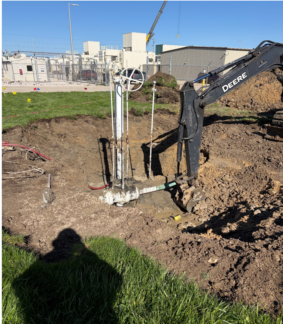
Excavation work to expose the old gas valve
