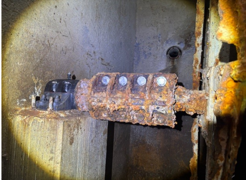
Recoated and refurbished submerged bearing housings, and replaced shaft coupling hardware
