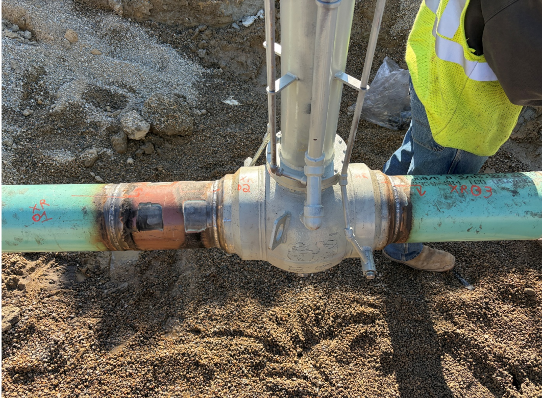
New valve after installation with X-ray and pressure testing passed
