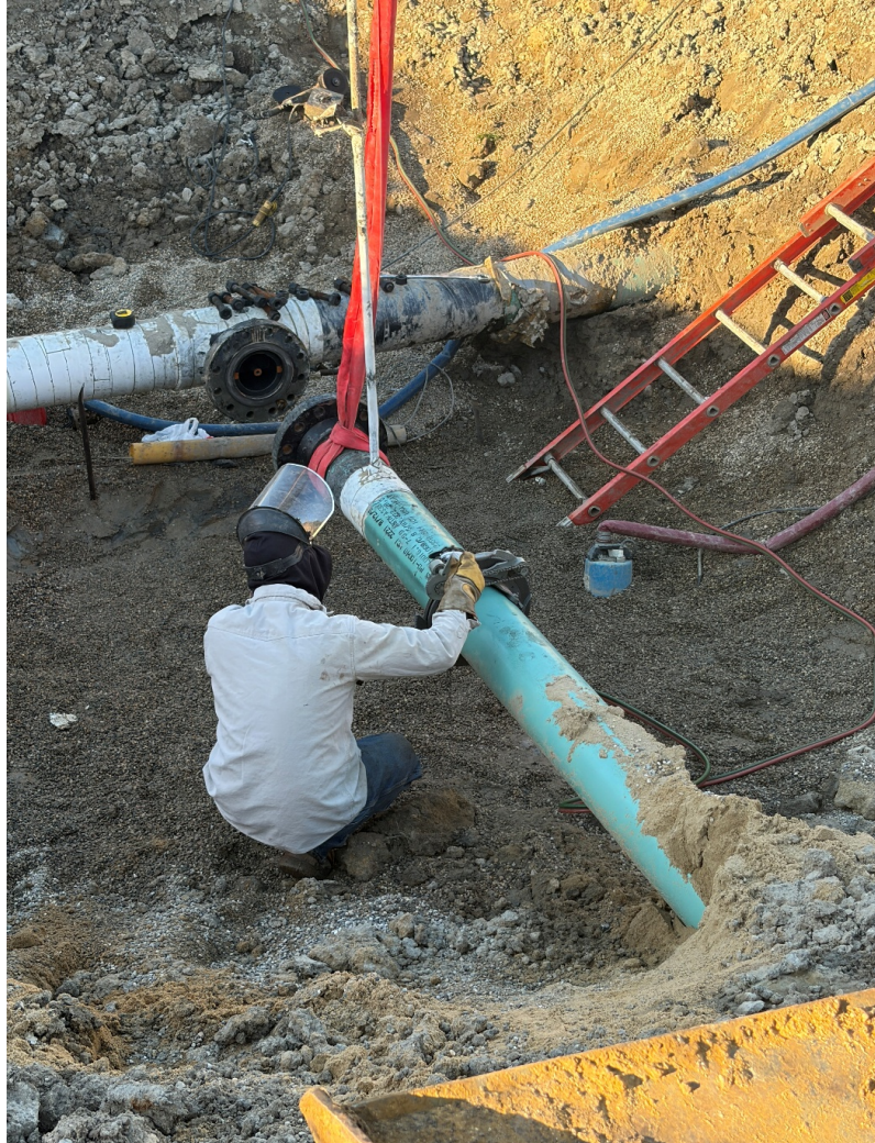
Verification of cut and rigging locations
