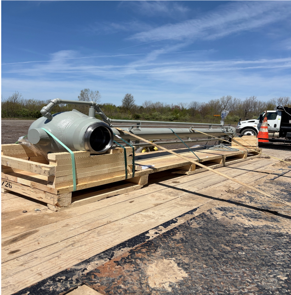
New gas valve arrival 1 week prior to construction
