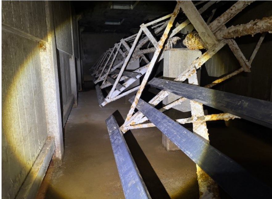
Replaced FRP paddles
