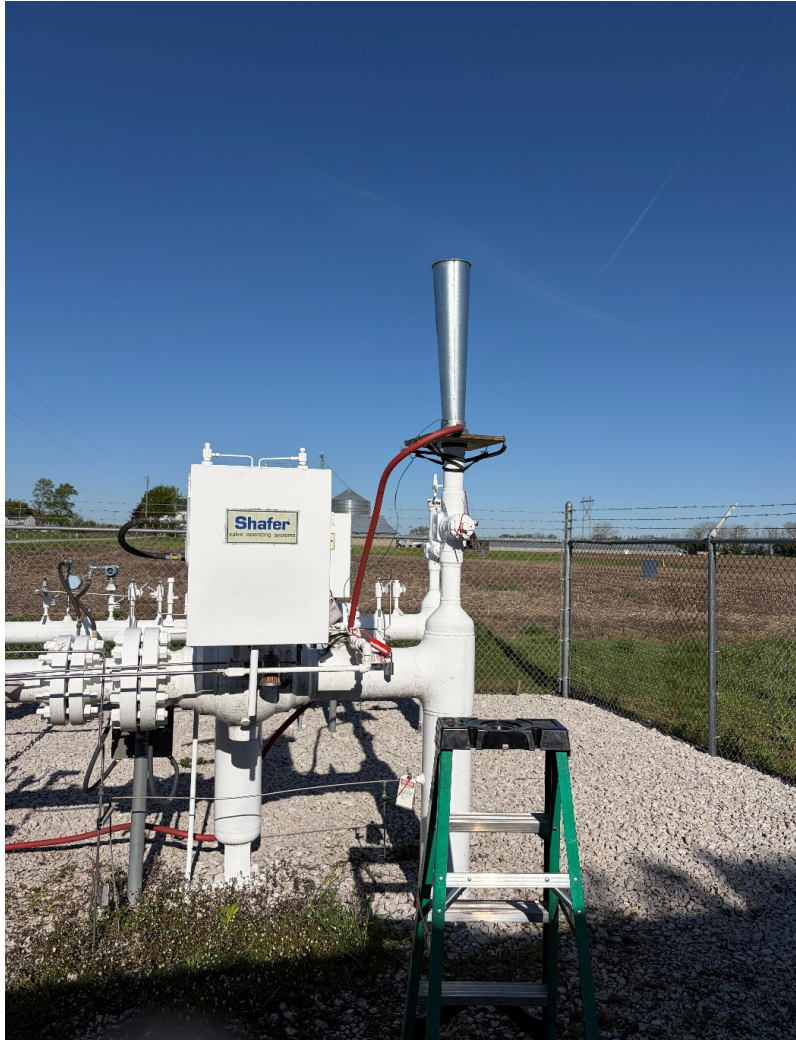
Air mover installation at Odorant Station
