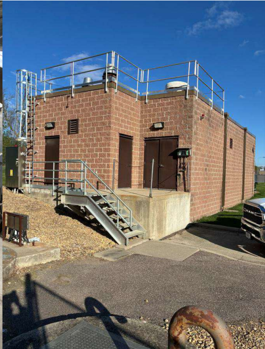
Courtland receiving station
