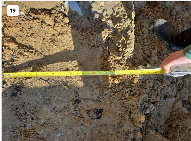
Sirocco Wall Footing Nominal 24 Inches Wide near Admiral Column Footing 1
