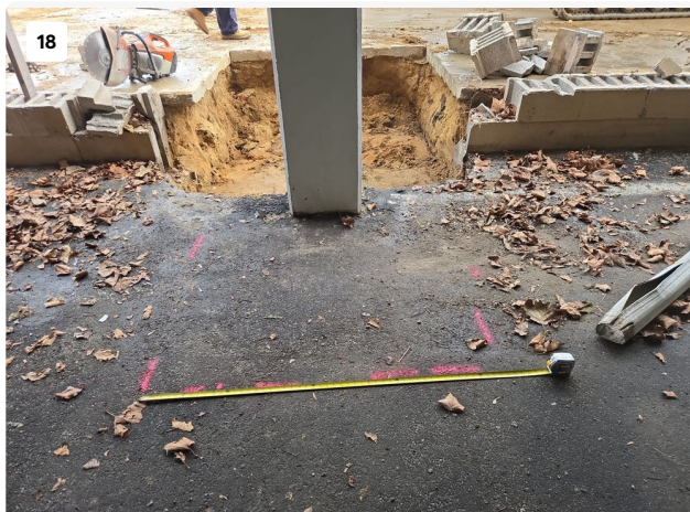
Column 2 Footing Width =Nominal 51 Inches Found by GPR Scan//Concrete Scan
