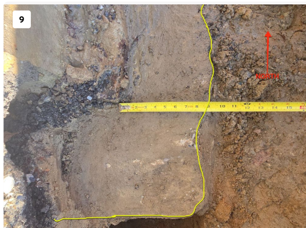
Column 1--Looking Down at Top of Footing Heel Footing Projection from Concrete Collar=Nominal 9 Inches
