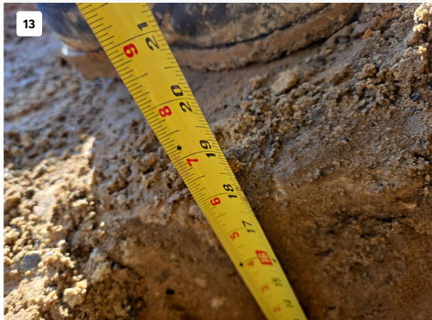
Column 1--North Face Footing Thickness=Nominal 19 Inches
