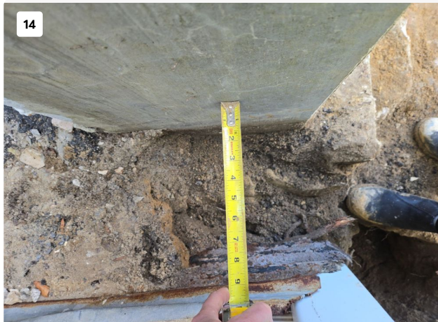
Column 3--Looking Down at Top of Footing Side (South Face) Projection from Precast Column=Nom- inal 7 Inches
