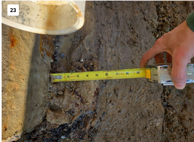
Column 1--Looking Down at Top of Footing Concrete Collar Around Precast Connection==Nominal 5 Inches Beyond East Face of Column
