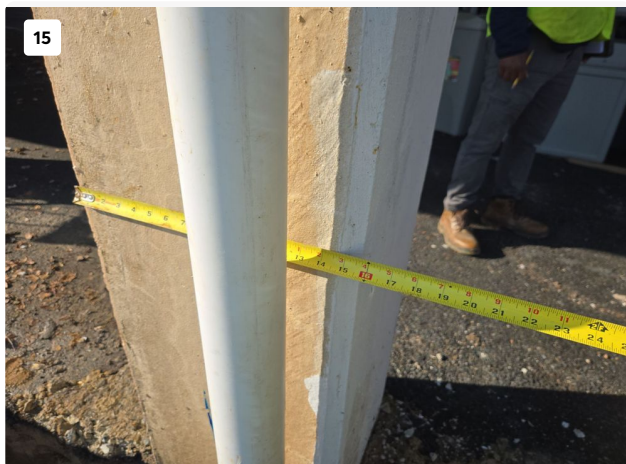
Column 1 Precast 16 Inch by 16 Inch Column
