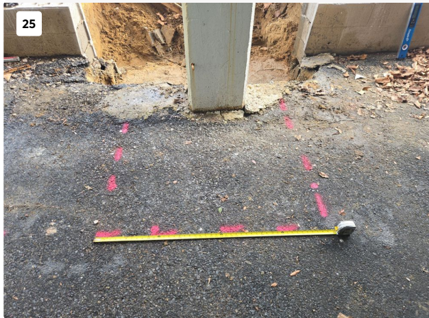
Column 1 Looking East Footing Width =Nominal 46 Inches Found by GPR Scan//Concrete Scan
