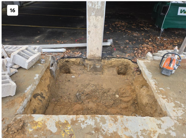
Column 2 Footing Width= 50 Inches Footing Length= 72 Inches Footing Thickness= 19.5 Inches (avg) Depth to Top of Footing= 16.5 Inches (avg)
