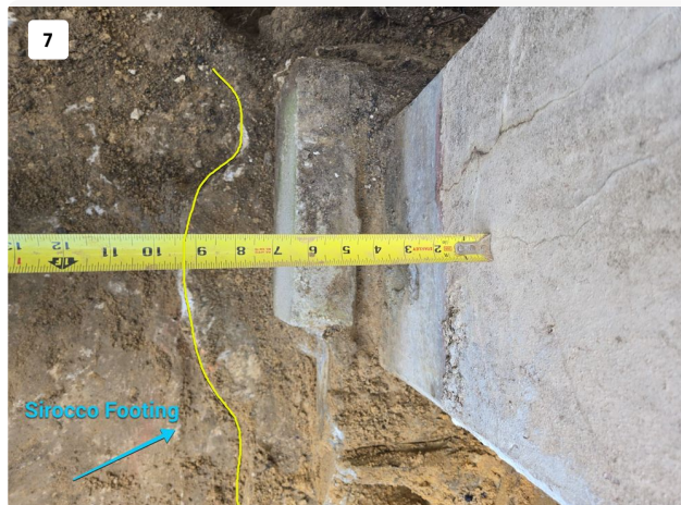
Column 3 (East Face) Looking down at top of footing Heel Projection Beyond Face of Column= Nominal 9 Inches
