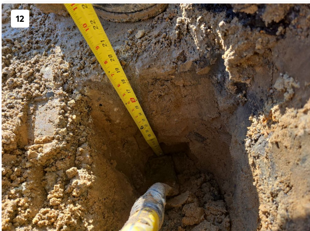
Column 1--North Face Footing Thickness=Nominal 19 Inches
