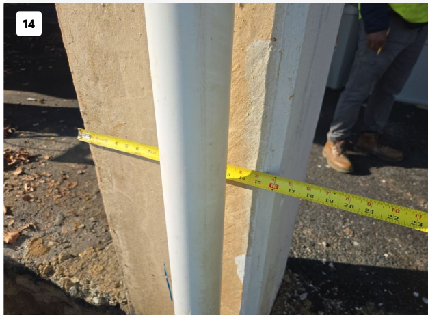
Column 1 Precast 16 Inch by 16 Inch Column
