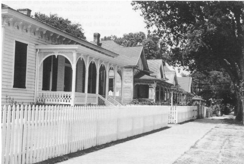
Ordeman-Shaw Historic District , Montgomery, Montgomery County, Alabama. Historic districts derive their identity from the interrelationship of their resources. Part of the defining characteristics of this 19th century residential district in Montgomery, Alabama, is found in the rhythmic pattern of the rows of decorative porches. (Frank L. Thiernonge, III)
