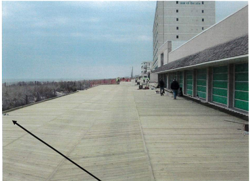
Light poles yet to be installed.
