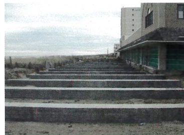
Rows of completed concrete beams.
