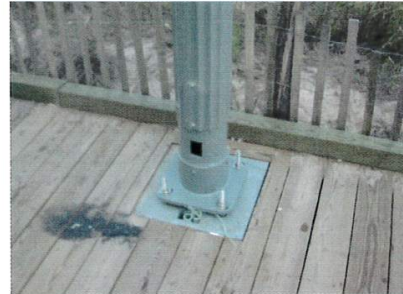
Composite light poles shown — one - piece shroud yet to be installed.
