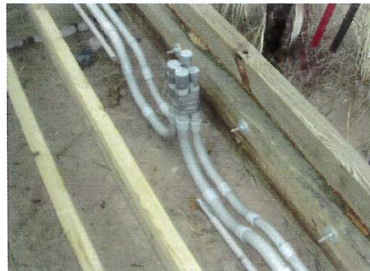
Conduit for 110V and low voltage to feed lights and future security cameras.
