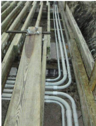
Conduit for 110V and low voltage to feed lights and future security cameras.
