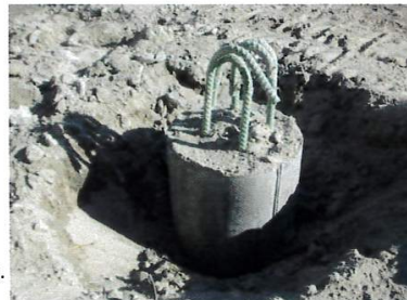
Completed cured piling.
