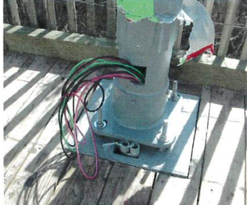
Composite light poles shown — one - piece shroud yet to be installed.
