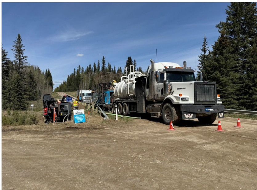
Conduit Installation - Horizontal Directional Drilling
