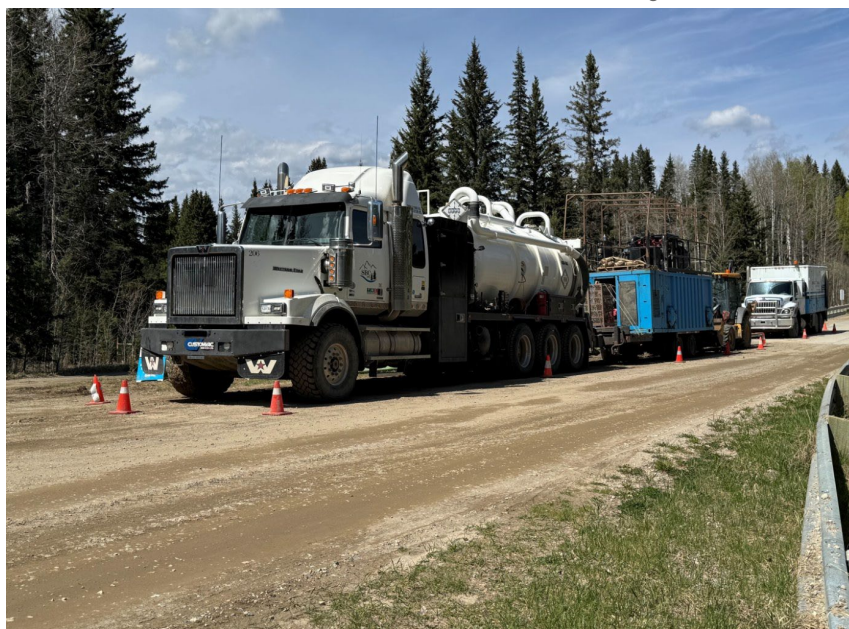
Conduit Installation - Horizontal Directional Drilling – Heavy Equipment
