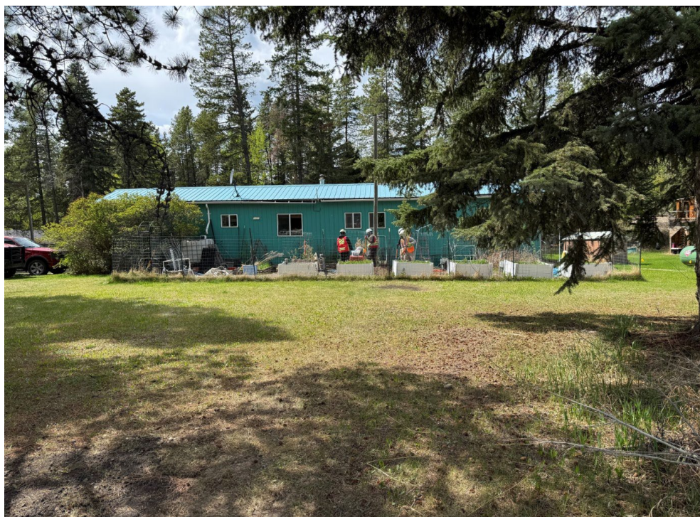
AFL Fibre Connect Installation
