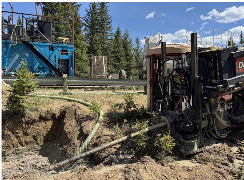
Conduit Installation - Horizontal Directional Drilling
