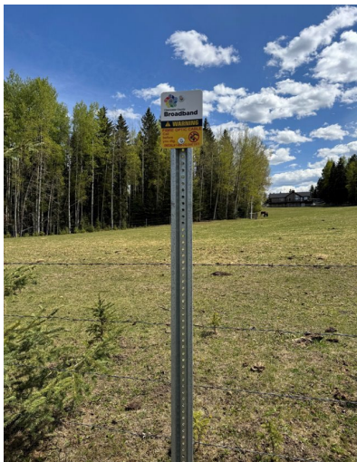
Clearwater County Network Marker Post
