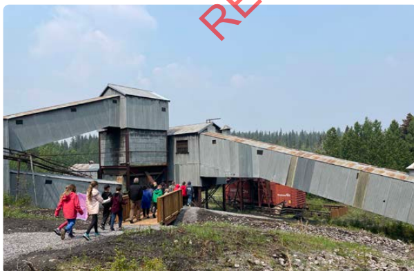
Brazeau Collieries mine site
