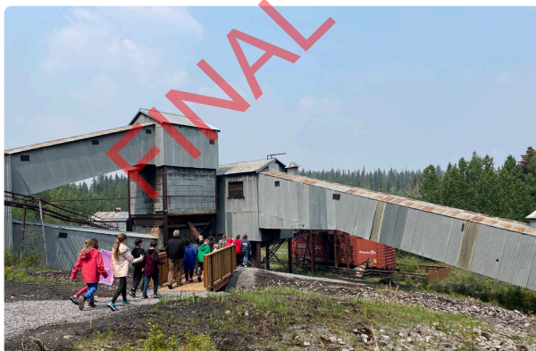
Brazeau Collieries mine site
