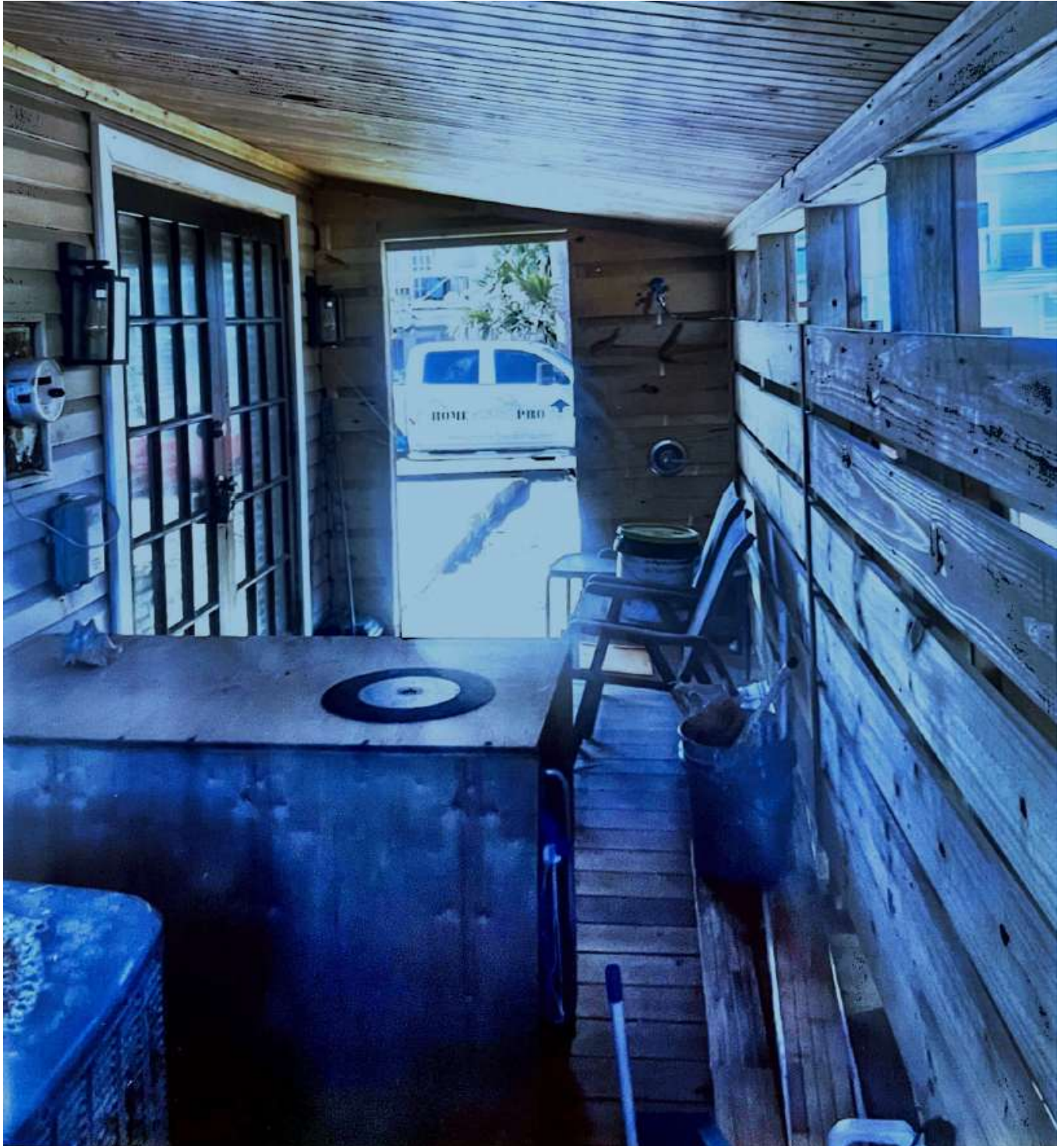
View of inside the porch structure
