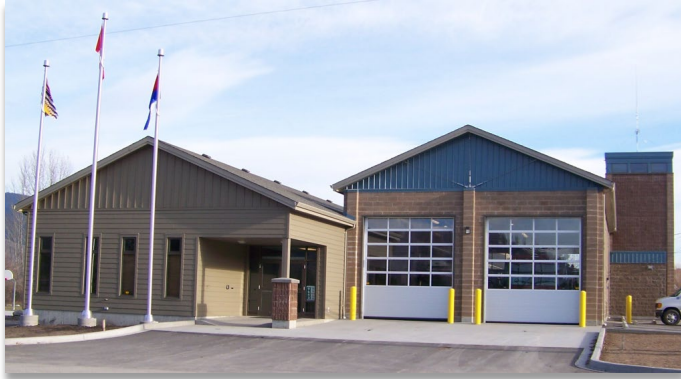
Lavington Fire Hall on School Road
