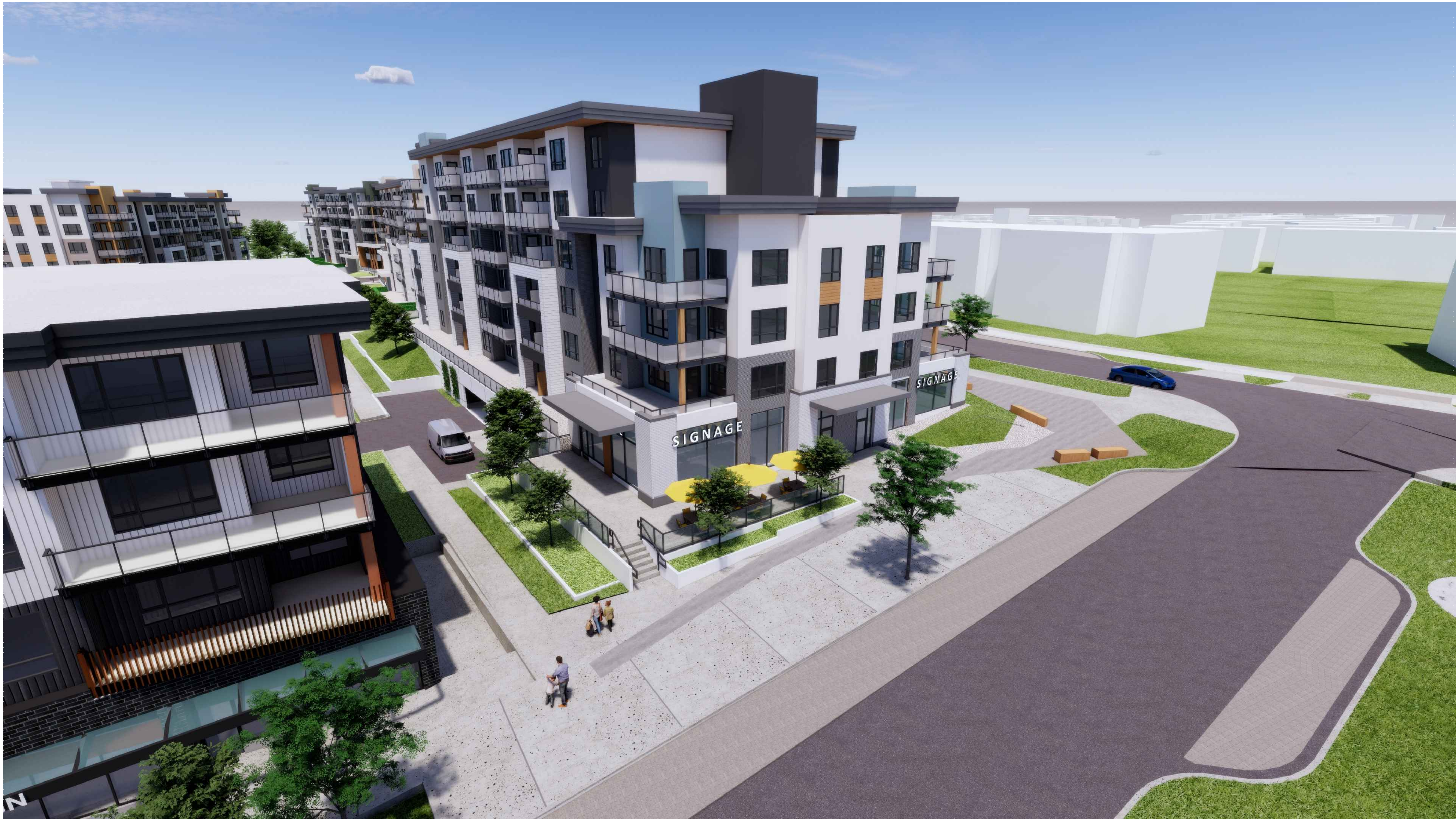
VIEW OF BUILDING E - NE CORNER VIEW OF BUILDING E - NW CORNER FACING ROYAL COMMONS ROAD
