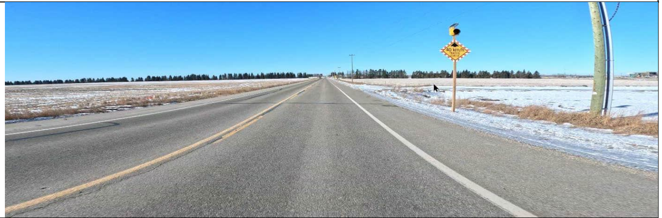
Approach View Looking East
