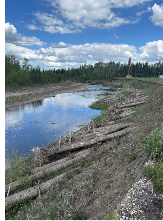
Red Willow Riverbank Stabilization
