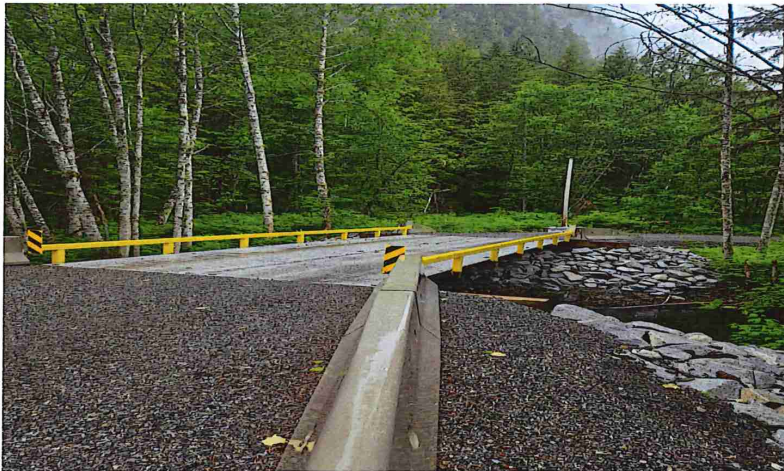
North Rainey Creek Bridge
