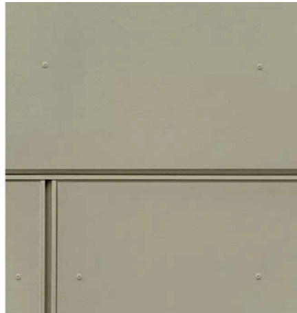
B.2.2: CEMENTITIOUS PANEL W/ COLOR MATCH REVEALS AND FASTENERS - LIGHT GREY
