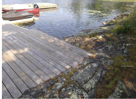
Photo 14. Dock 2 platform shaped to bedrock.
