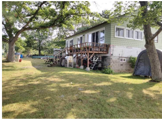
Photo 8. Western wall of existing dwelling with existing deck.
