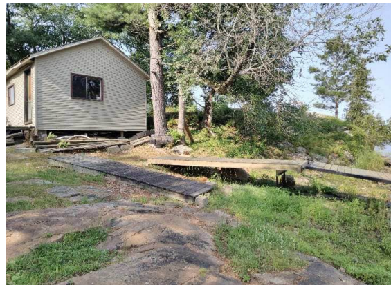
Photo 18. Existing accessory structure to north side of property; platform to Dock 1 (pinned to bedrock).
