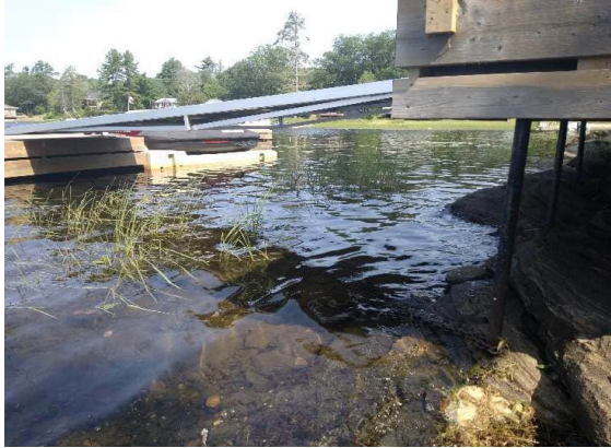
Photo 13. Dock 2 platform pinned to bedrock.
