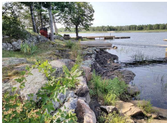
Photo 12. Western shoreline frontage; facing south toward Dock 2.
