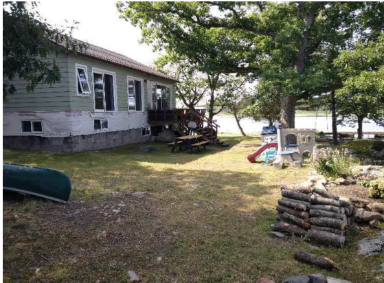
Photo 21. Western wall of existing dwelling; location of proposed new deck.
