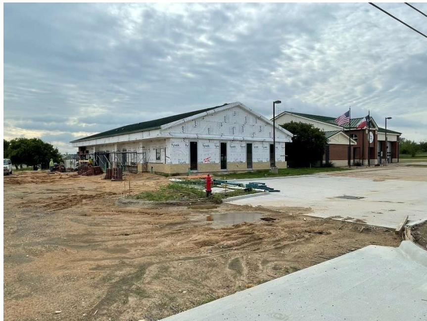
Haslet Fire Station Improvements
