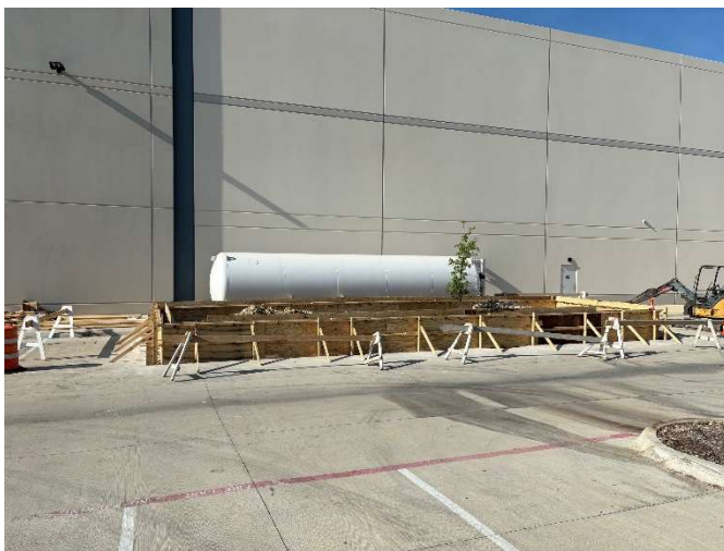
CTDI Haslet – 405 Westport Parkway- interior work currently underway. CO2 Tank has been installed on south side and connected to building. Generator installation has started on east end of building.
