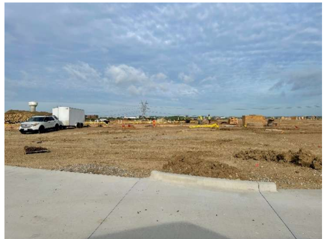
Infrastructure for Freeman Toyota being installed.
