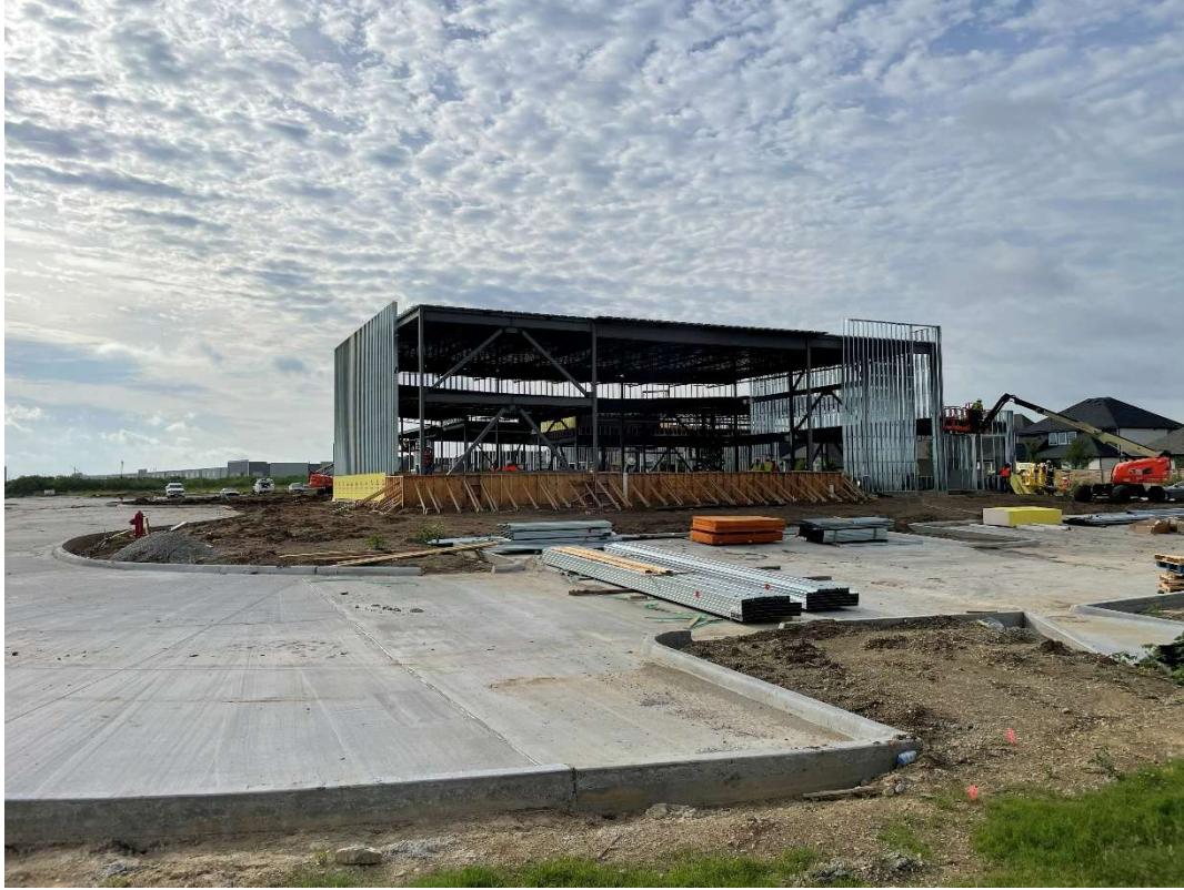
Cross City North Church Site Work Haslet Parkway at Sweetgrass Blvd.
