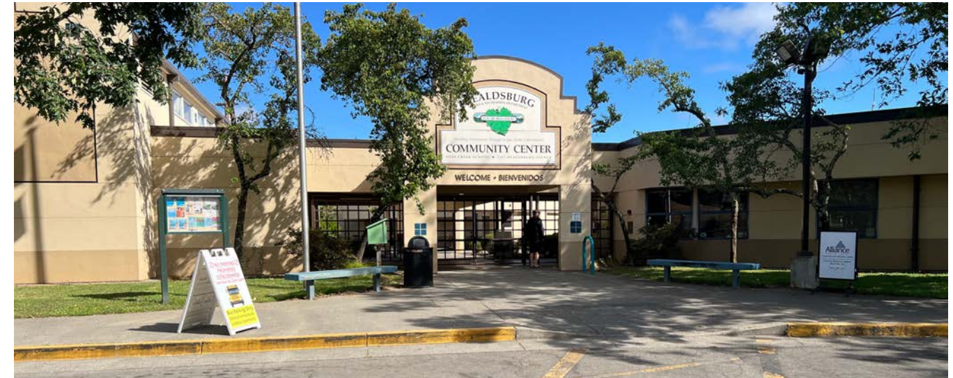
Area 1: view of entrance on north side of central campus, looking south.
