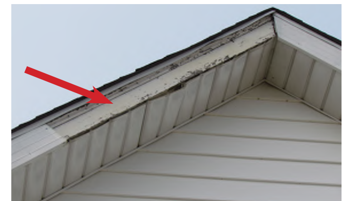
Painted wood trim will be replaced in kind.
