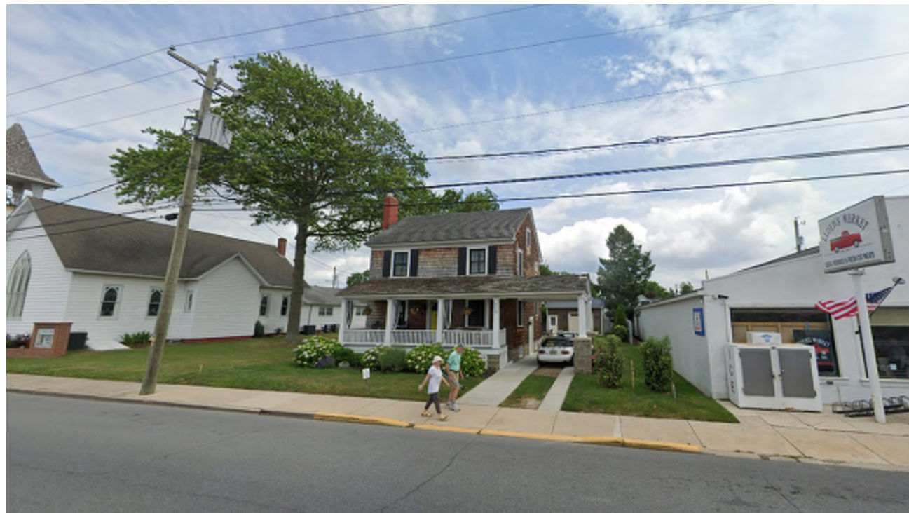
609 Savannah Rd, Existing west elevation of the Church
