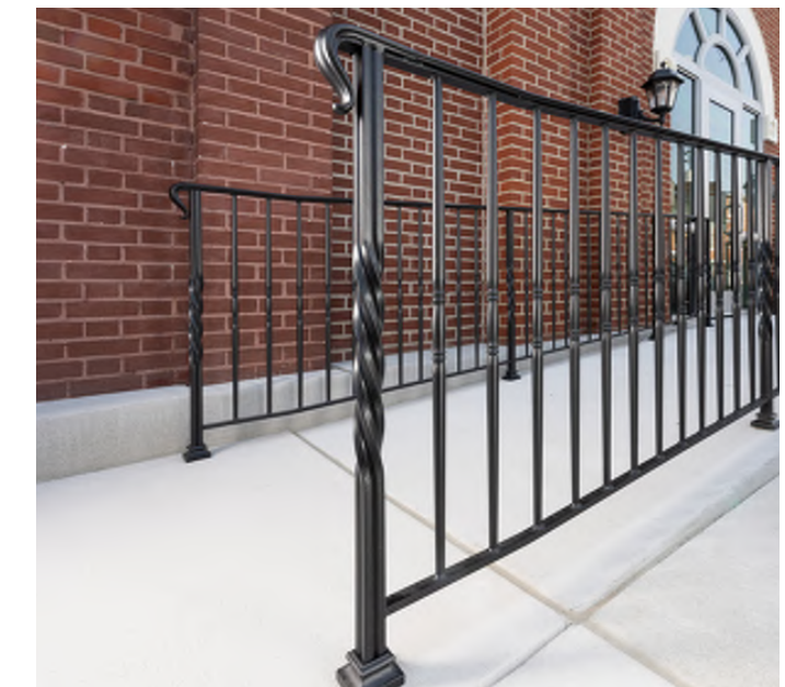
Typical exterior railings are steel, painted black.
