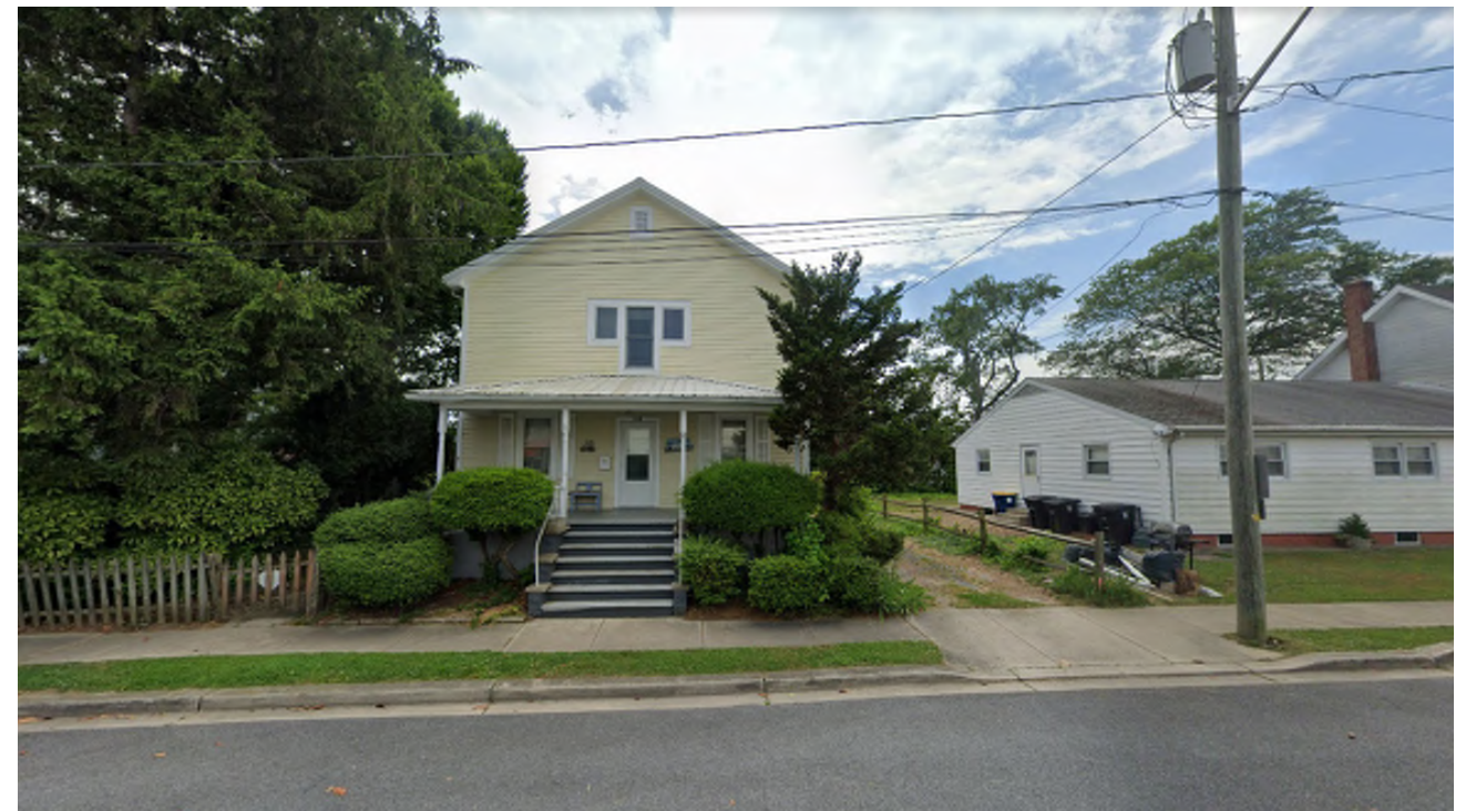
Neighboring Property at 108 Dewey Ave, Existing south elevation of the Church
