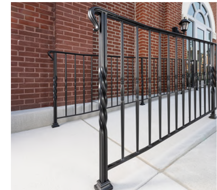
Typical exterior railings are steel, painted black.
