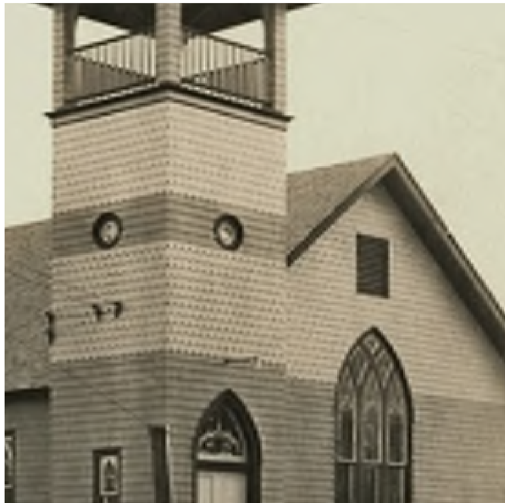
Church's original two-tone shingle siding, with dark trim, will be recreated.
