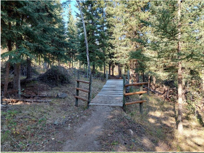
Figure 16 This cattle fence crossing on the Mimi Falls Trail does not feature a handrail and has a significant fall height on the downhill side. The sloped wooden surface is slippery in wet and icy conditions.
