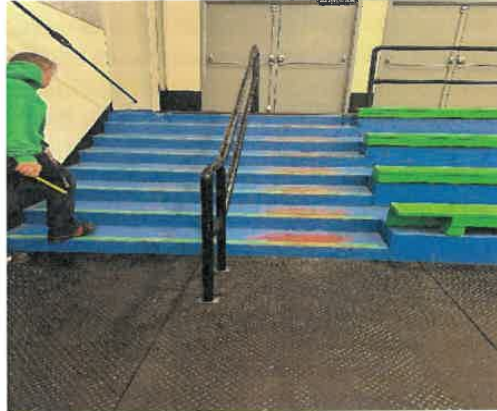
Figure 4: Lift work area
