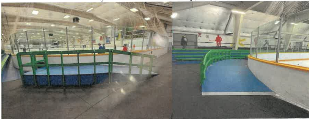
Figure 1: Current accessible viewing platform
