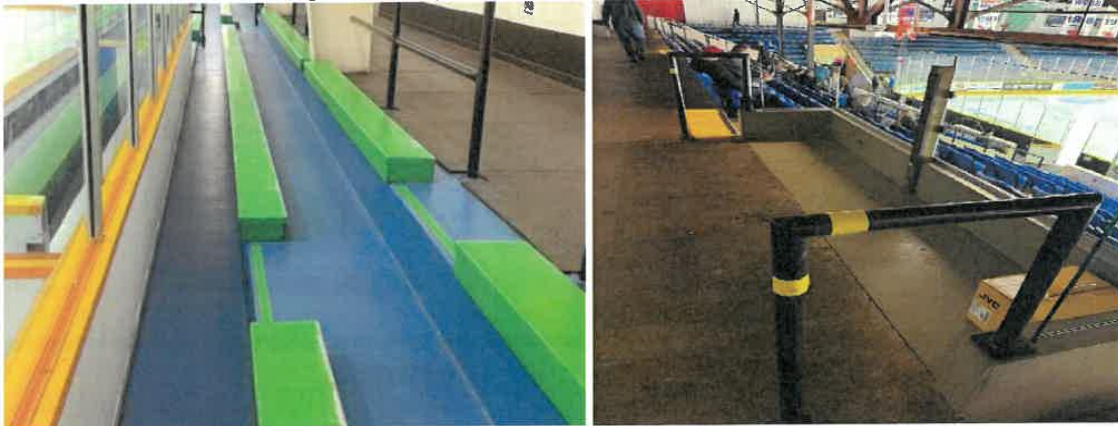
Figure 5: Viewing platform location and example of similar areas in other arenas
