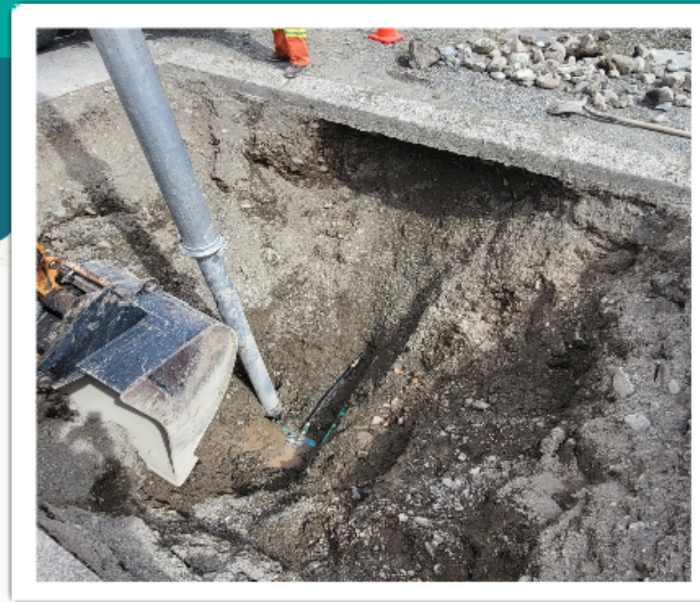
SHUTOFF VALVES REPLACEMENT
