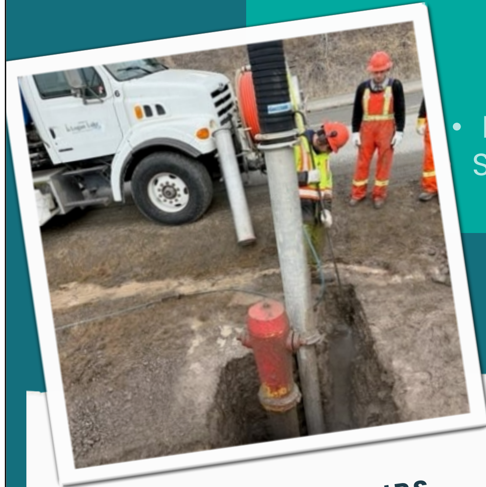
HYDRANT REPAIRS
