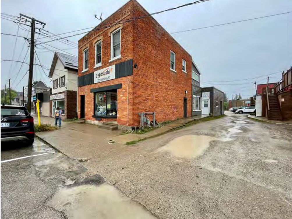
ADJACENT PROPERTY AT 16 TROWBRIDGE STREET WEST – c.1860 brick commercial building
