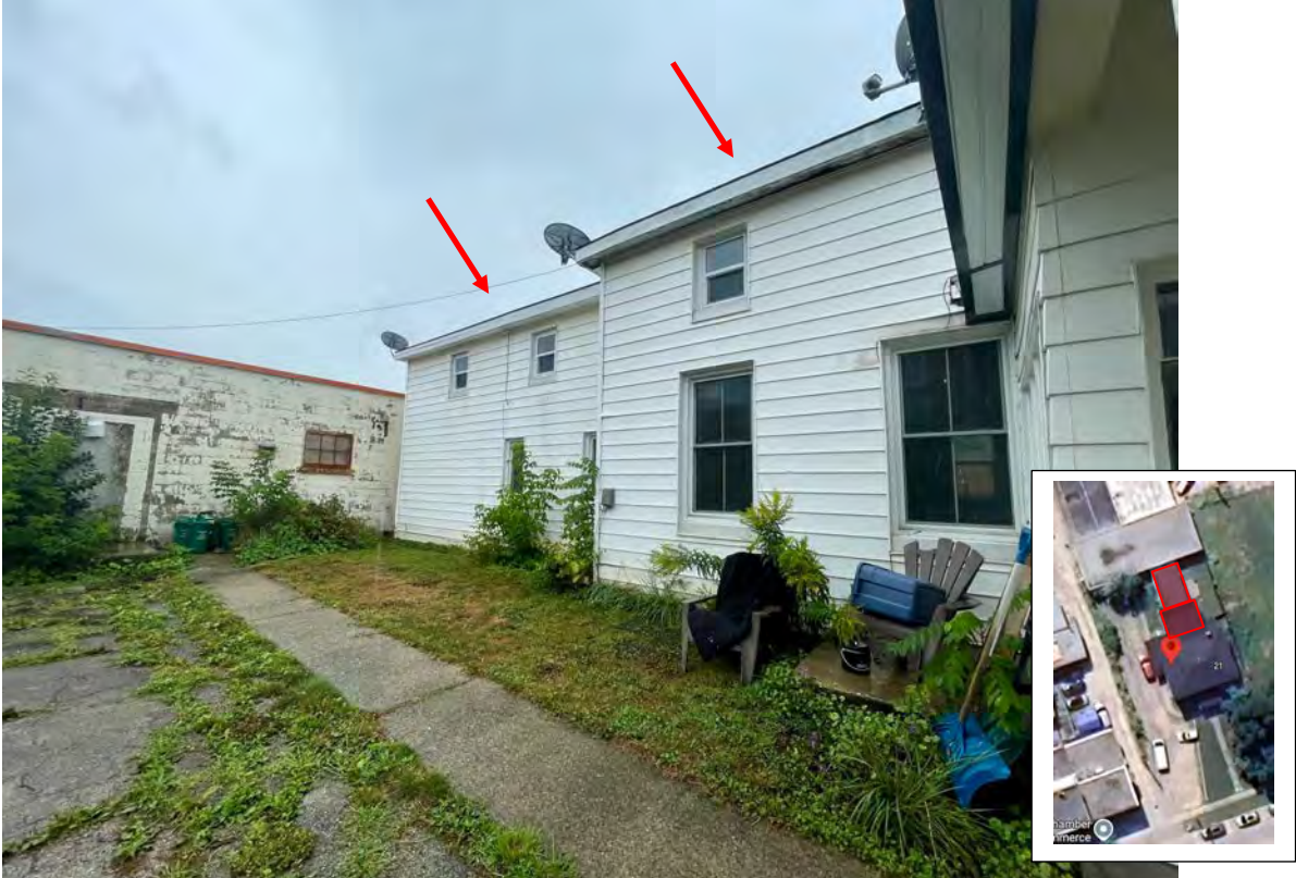
19 NELSON STREET WEST, REAR ADDITIONS – the rear additions are different heights and are clad in vinyl
