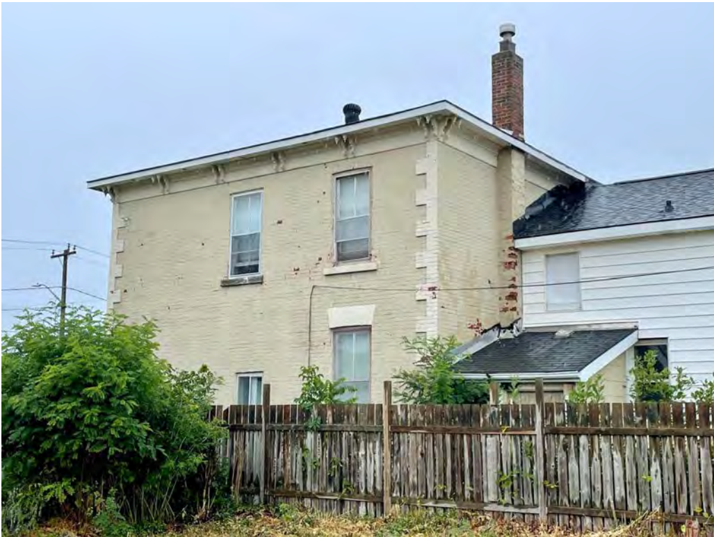
19 NELSON STREET WEST, WEST SIDE ELEVATION – raised brick corner quoins and paired brackets in the roof cornice – windows have brick jack arches and wood sills – no original chimneys
