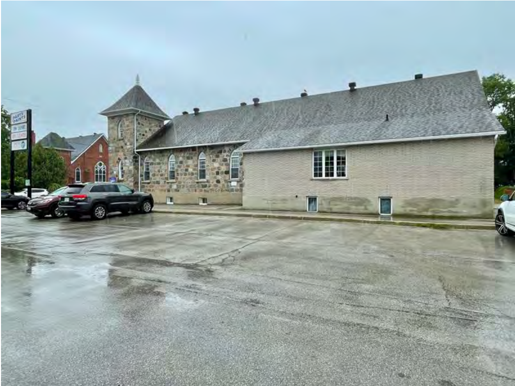
ADJACENT PROPERTY AT 34 TROWBRIDGE STREET WEST – c.1925 fieldstone church
