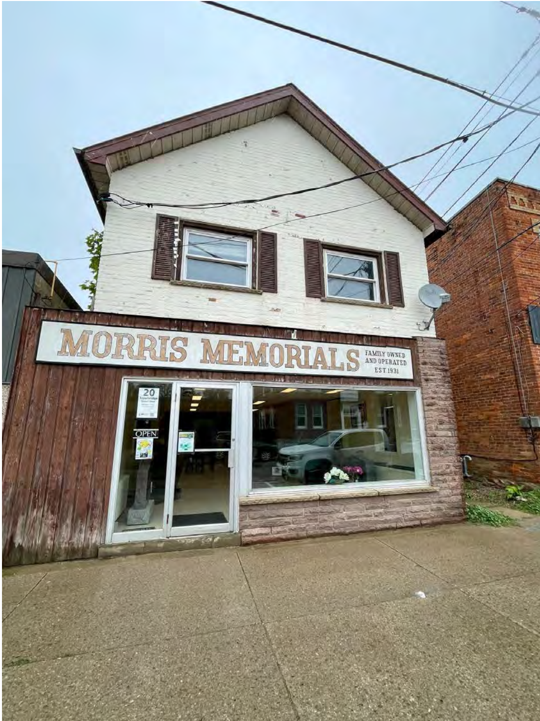
20 TROWBRIDGE STREET WEST – 2-storey brick commercial building with a front facing gable
