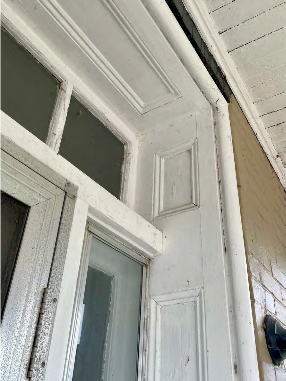
19 NELSON STREET WEST, FRONT ENTRANCE – original paneled door surround
