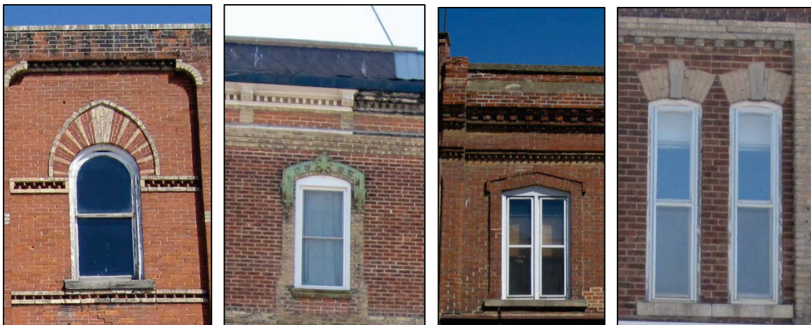
Window openings are important to the architectural character of buildings.
