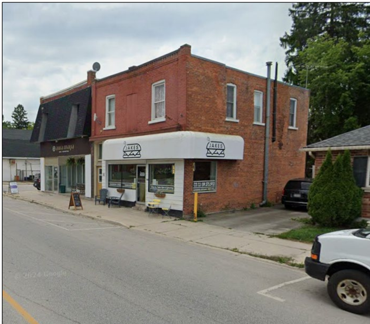
Figure 3: Front and Side View (Google Streetview image)
