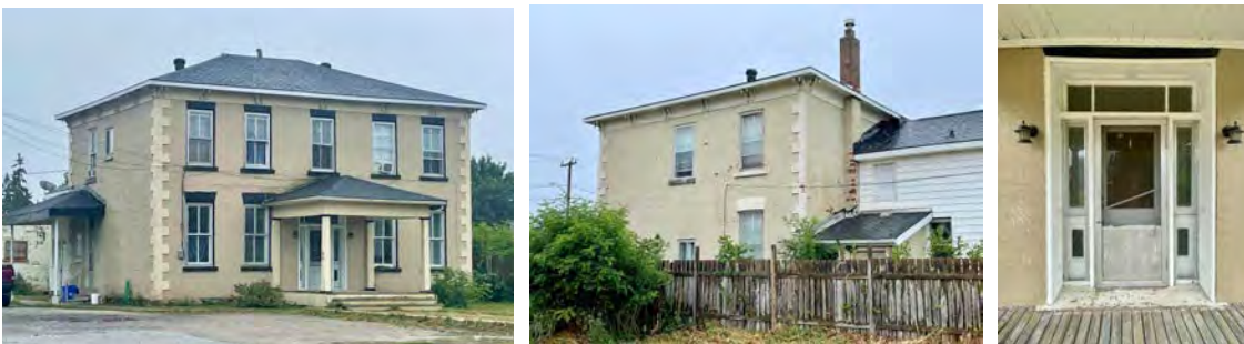
19 NELSON STREET WEST: 2-storey, 5-bay, brick dwelling that has been heavily altered and is in poor condition
