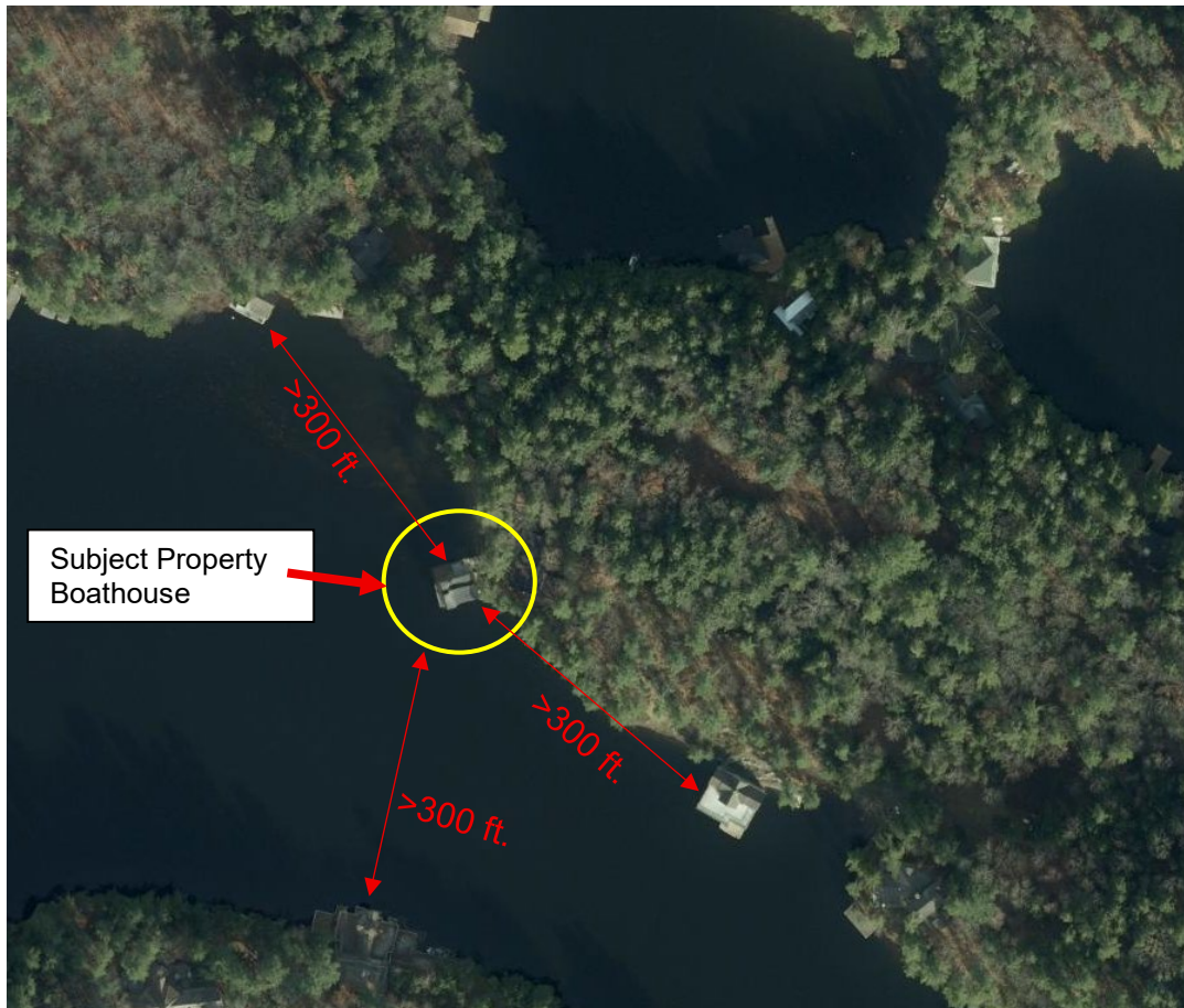
Figure 2: Aerial view of the existing boathouse and neighbouring properties.
