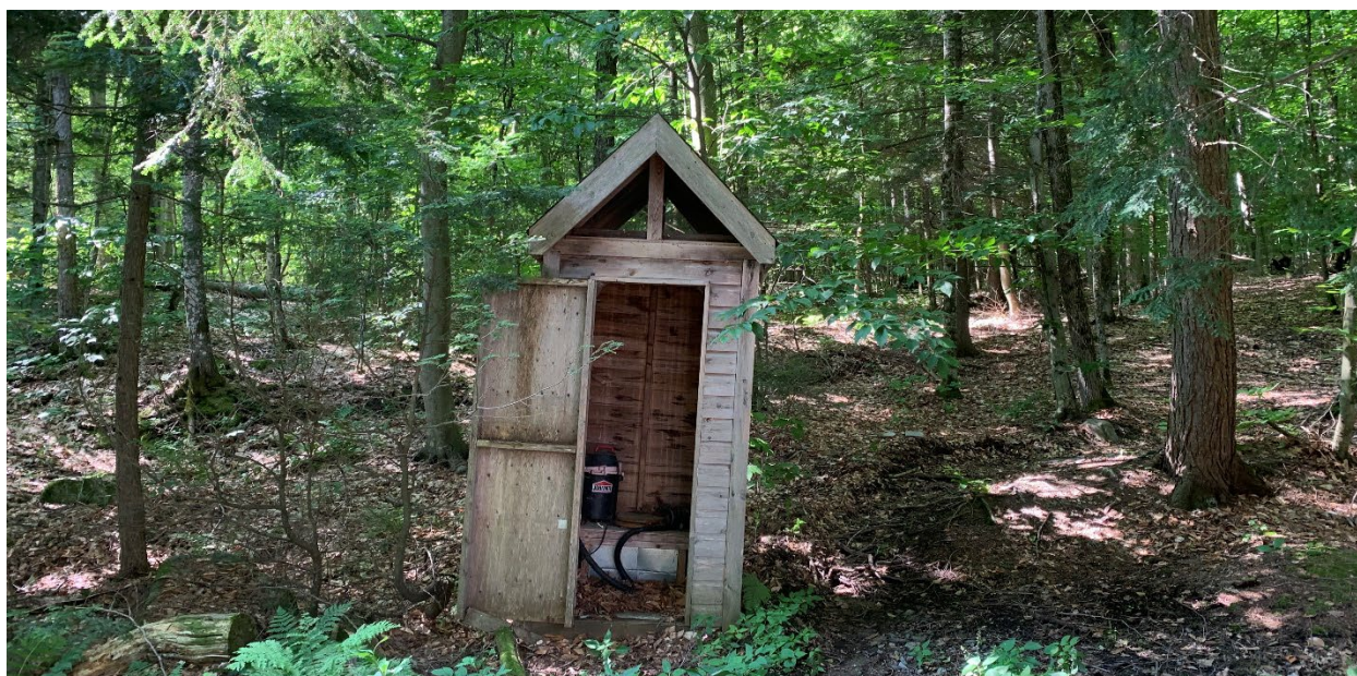
Figure 5: Pumphouse on the Benefitting Lot.
