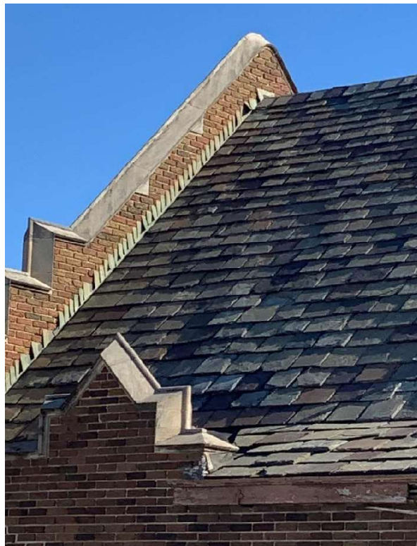
Figure 2 - Slate Tile Roof
