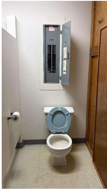
Figure 14 - Panel in Toilet Stall
