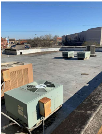
Roof: Roof top equipment appear to be properly flashed weather tight
