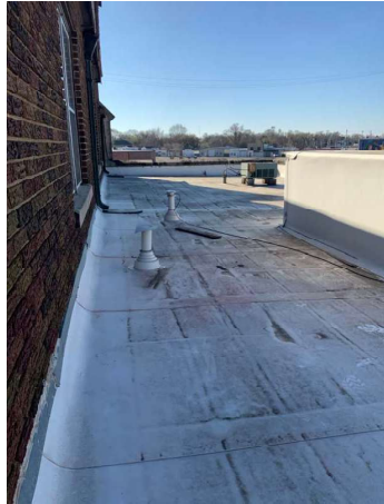
Roof: TPO roof membrane in good condition
