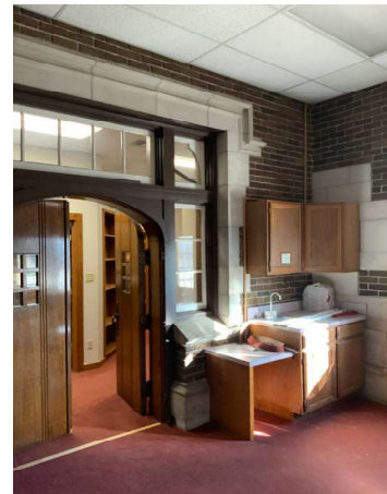
First Floor: Historic details remain in good condition
