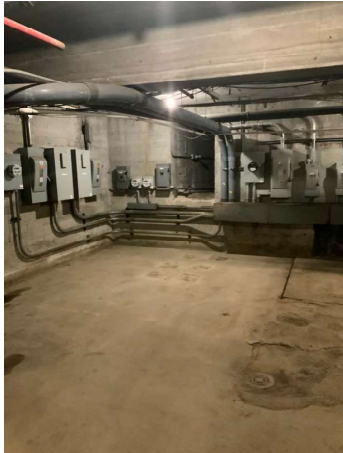
Basement: Dry basement at electrical and equipment rooms
