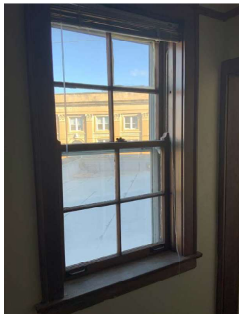
Building retains historic windows and in operable condition
