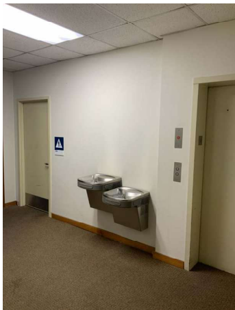
First Floor: Restrooms and other ADA accommodations provided on first floor only
