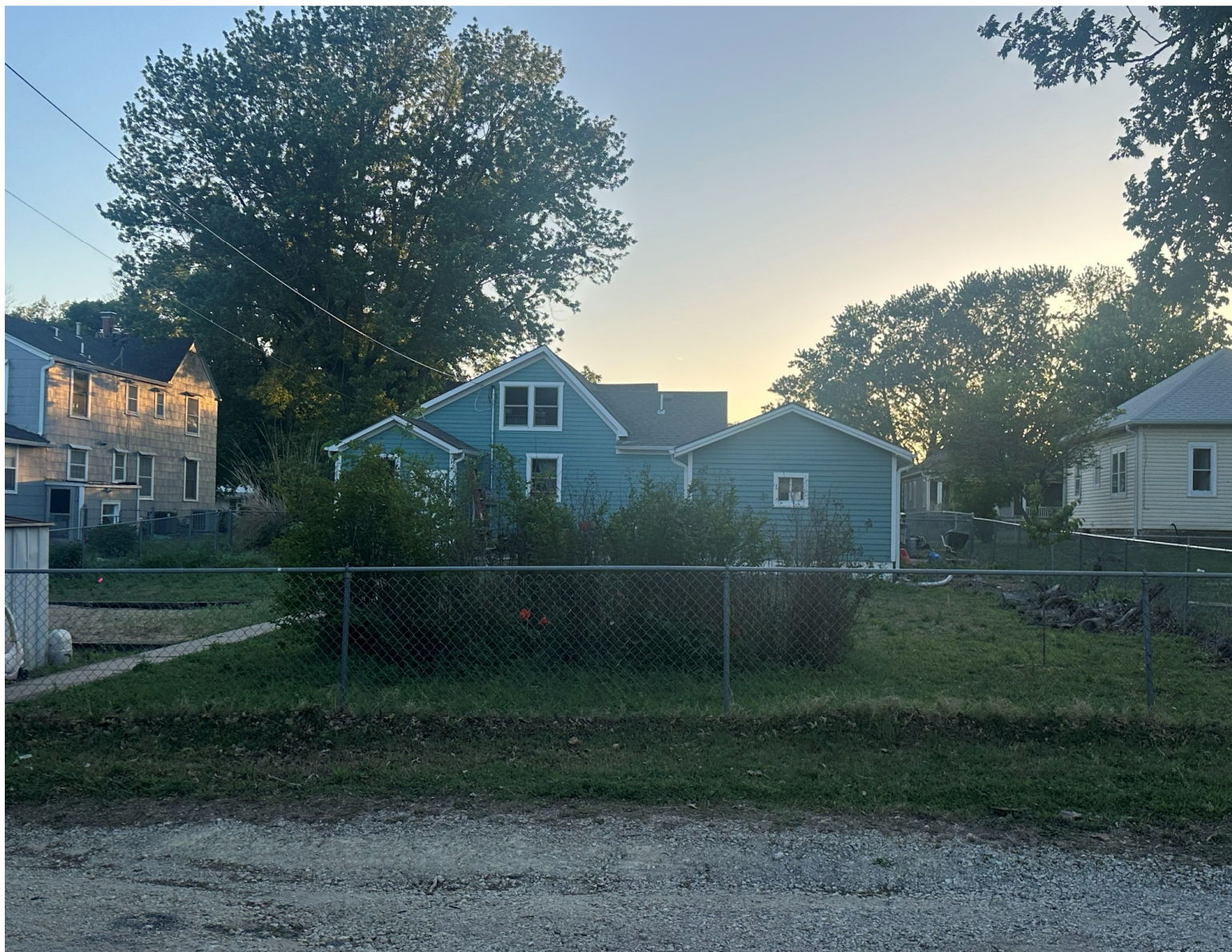
View from across East alley
