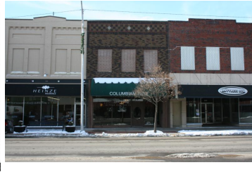
511 N Main St. Principal elevation. 01/12/2011. Payne, Glen.
