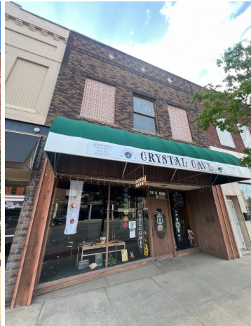
511 N Main St. 511 N Main St. East elevation. C. Ammerman 05/2024
