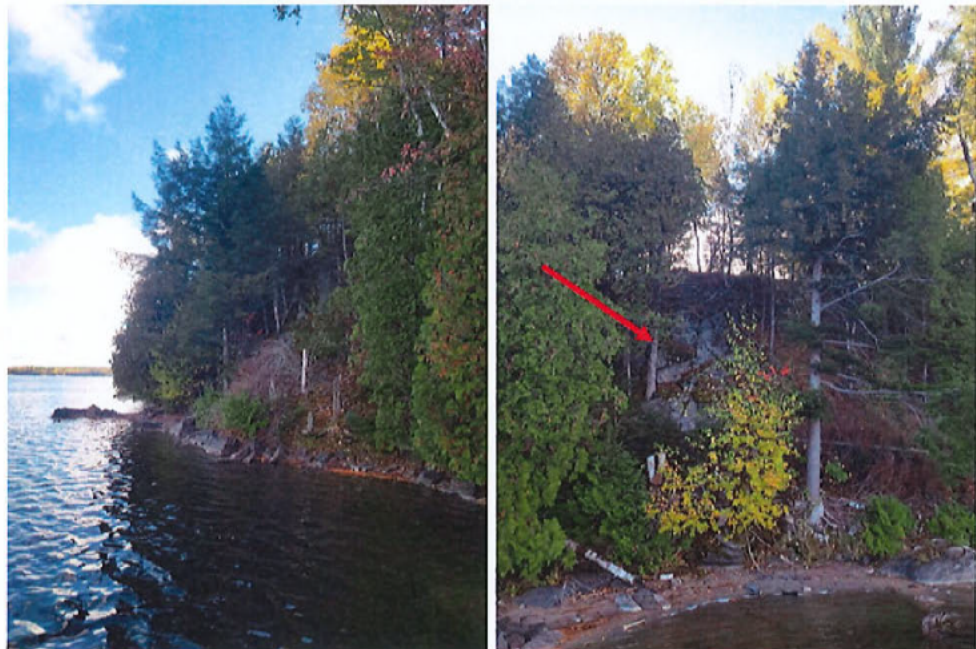
Photo 8 General view of side slopes, parking spots on top, October 2023.
