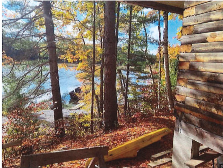
Photo 5 Middle of Front Slope, downwards view, October 2023.
