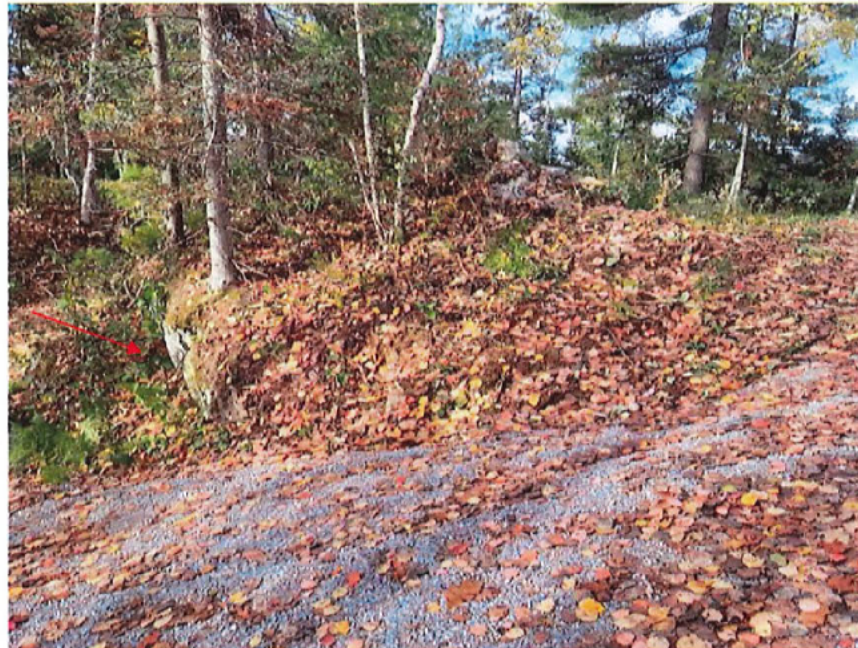
Photo 2 Top of front slope, side view, October 2023.
