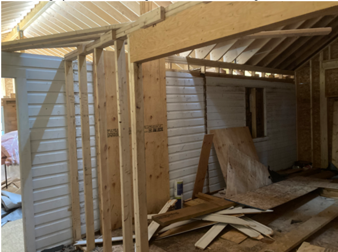
Figure 2. Photo from the interior of the existing dwelling showing the outside wall on the southwest of corner of the house has been enclosed by new development.
