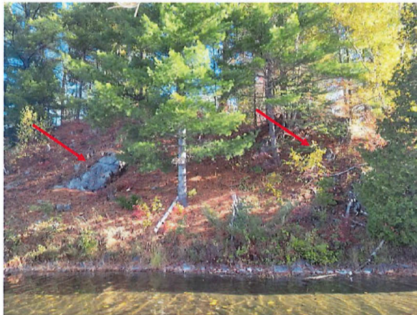
Photo 6 General view of back slope, parking spots on top, October 2023.
