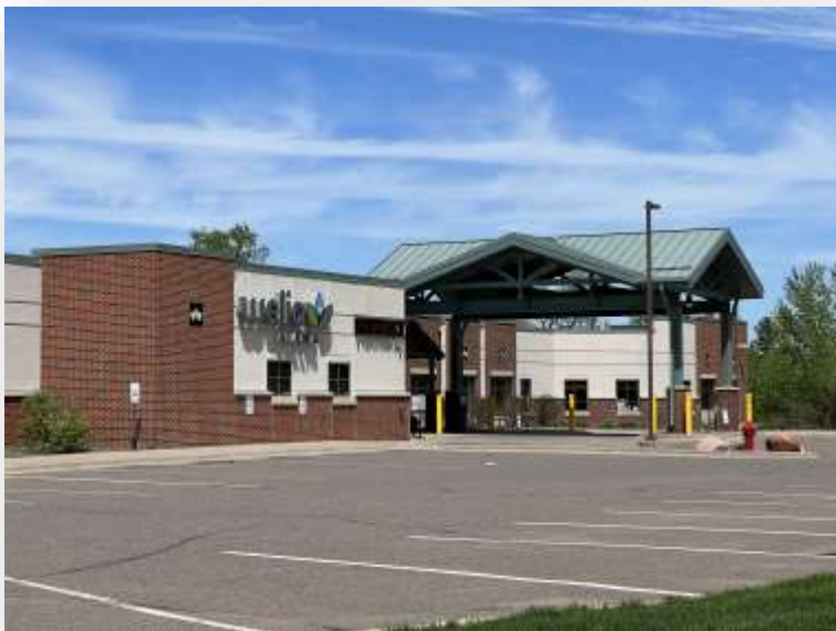
(Above) Welia Health is a major Pine City service and amenity, and is one of the major features of the Northridge neighborhood, which also includes a retail mall, an auto dealership, and the Pine County Courthouse, as well as several multi-unit residences including Timber Pines.
