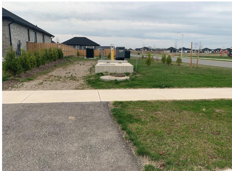
Figure 7 – Errol Woods Pump Station Site
