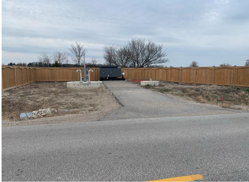
Figure 8 – Egremont Estates Pump Station Site
