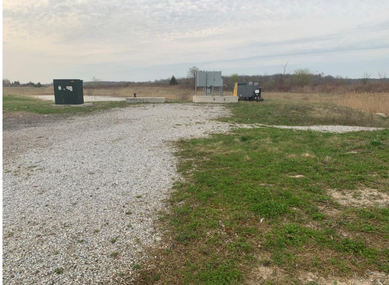
Figure 6 – Radcliff (Silver Springs) Pump Station Site
