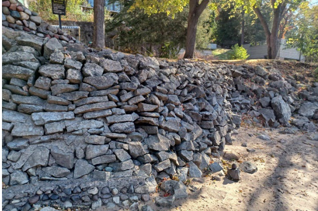
Figure 6 Limestone wall with no mortar
