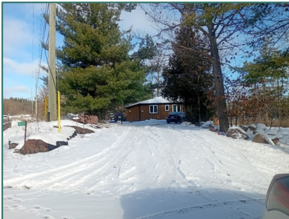
Photo 2 Driveway to proposed severed lot (existing secondary dwelling)
