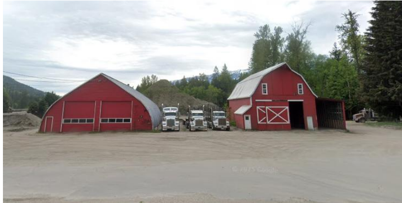
Figure 3: Existing accessory buildings on site
