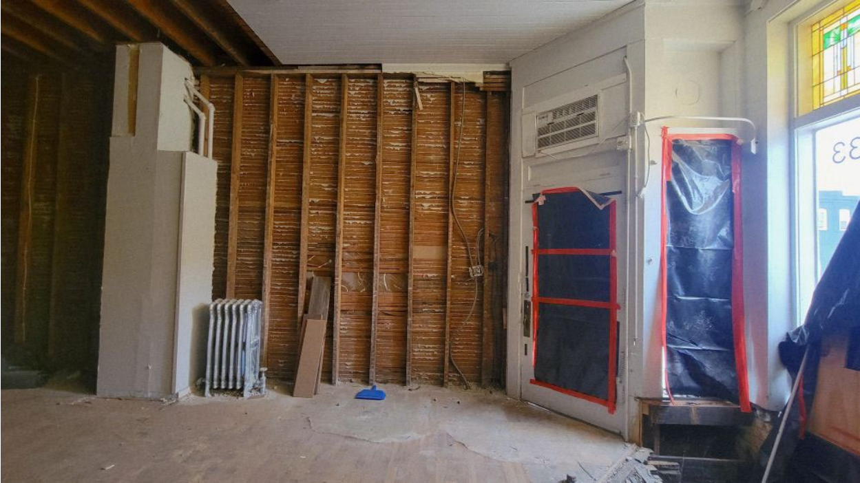
1233 Milwaukee Interior Storefront Space, current conditions
