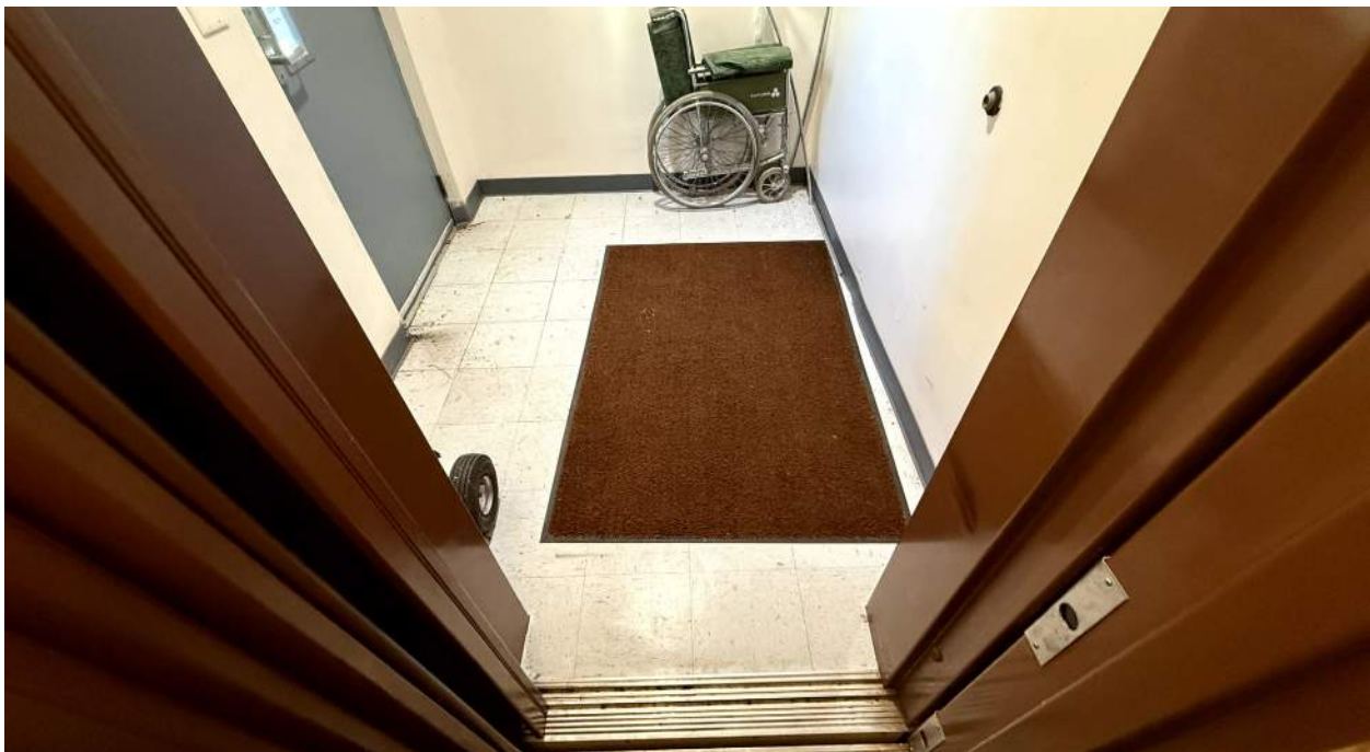
Elevator lobby, lower level. Exterior elevator lobby door.
