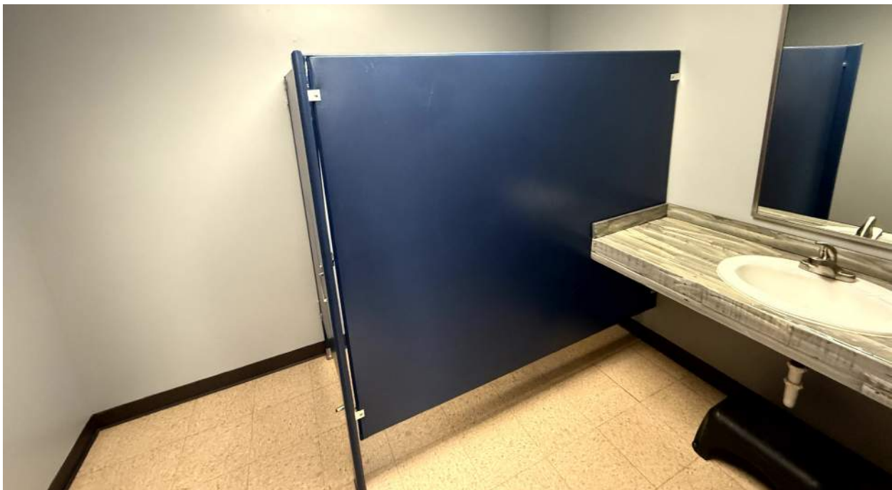
Accessible restroom , upper floor.
