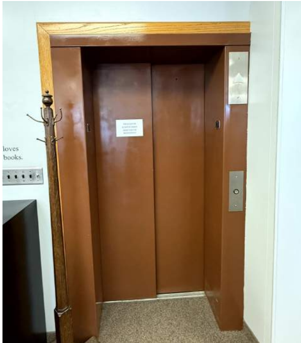
Elevator, upper floor.
