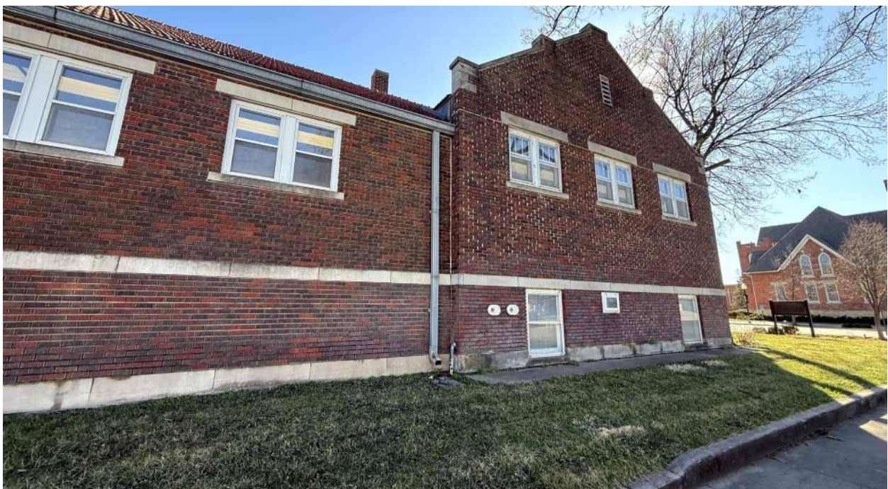
North exterior wall, original 1917 construction and 1982 addition
