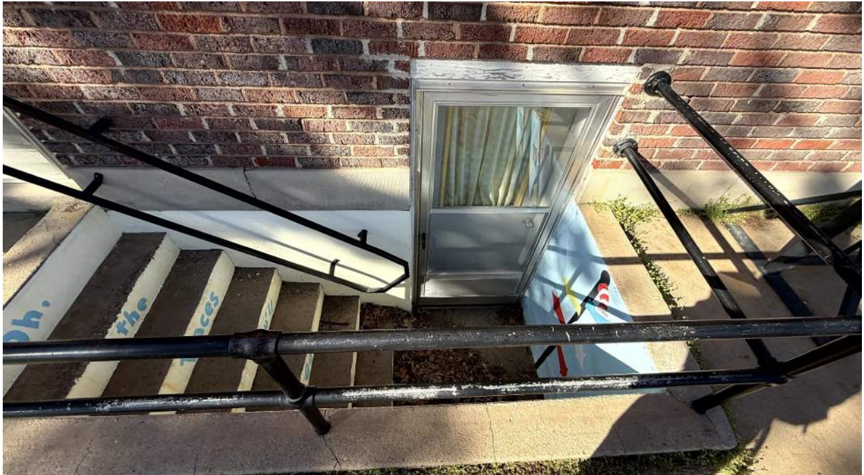
South exterior wall, lower floor reading/activity room entrance, original 1917 construction
