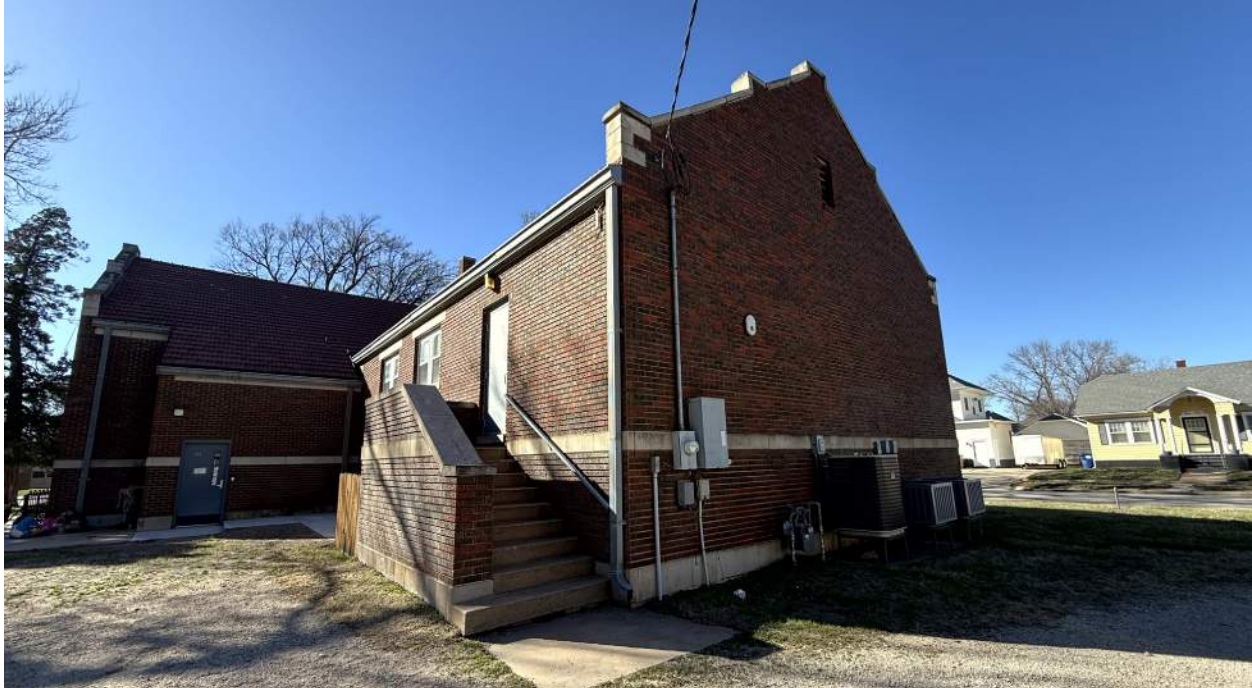
Southeast exterior wall and exit stair, 1982 addition
