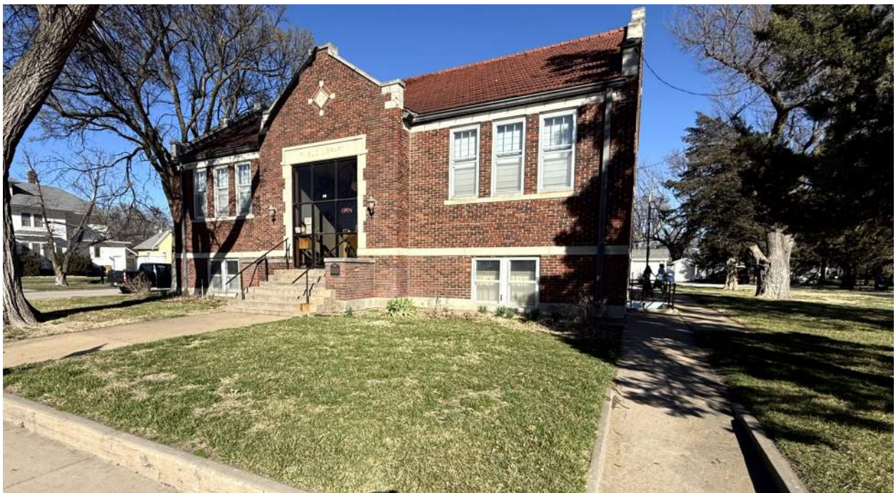
West exterior wall, original 1917 construction. Sidewalk to lower level entrance
