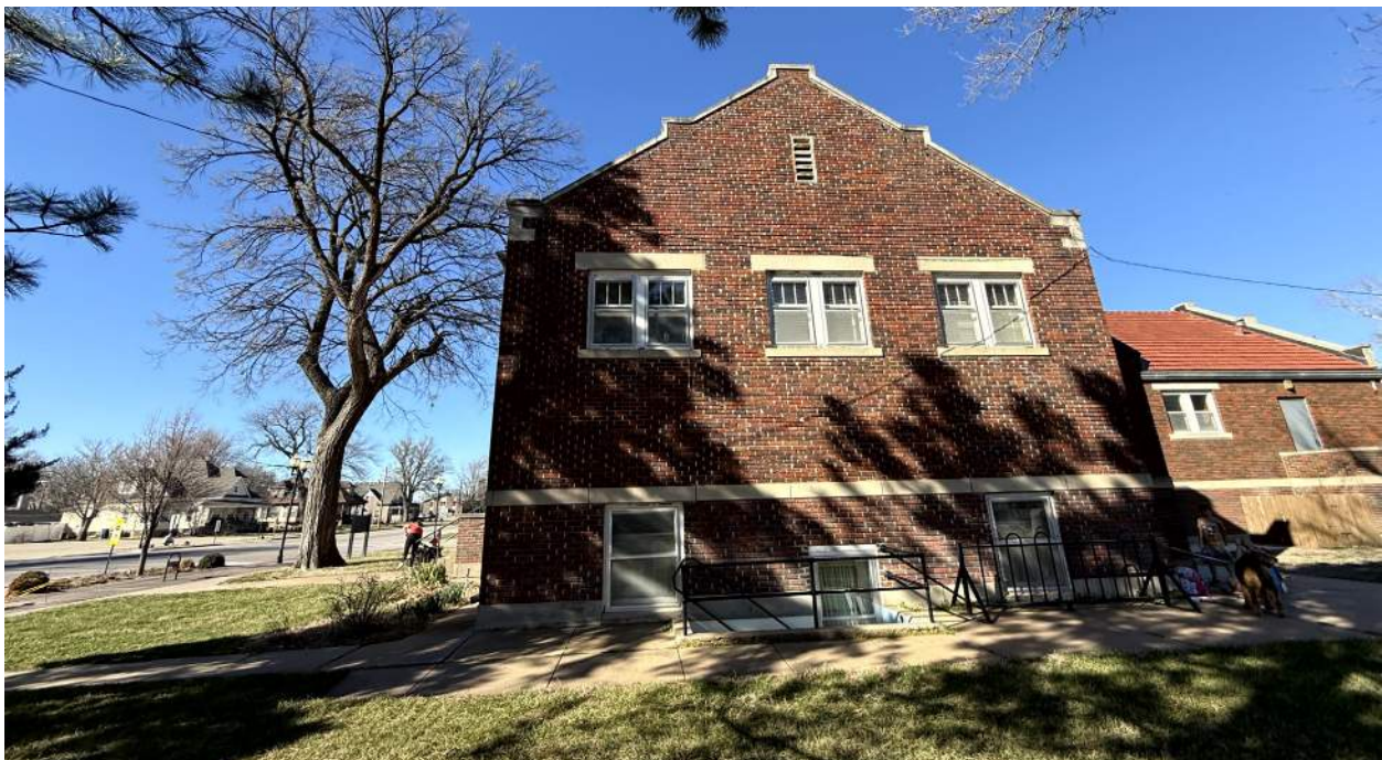
South exterior wall, original 1917 construction.
