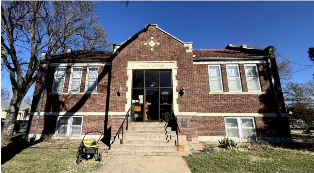
West exterior entrance, original 1917 construction
