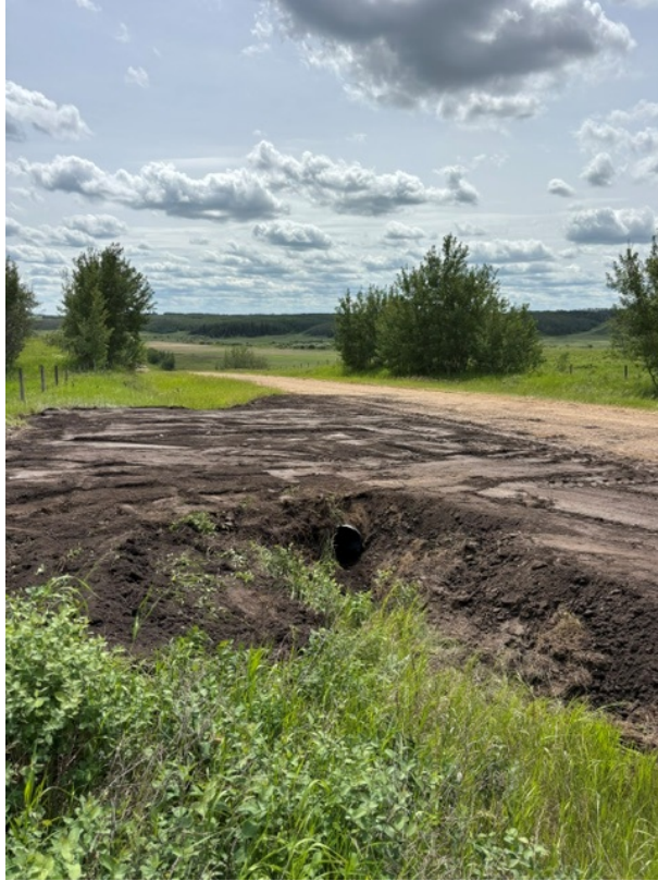
Public Works Figure 6.02. New Approach Install
