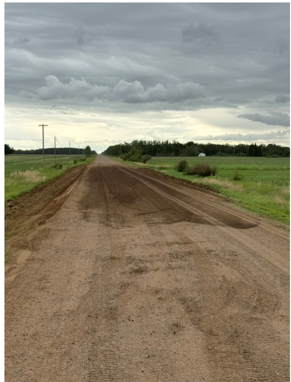
Public Works Figure 2.01. Road Patching Work with 1-1/2" Material
