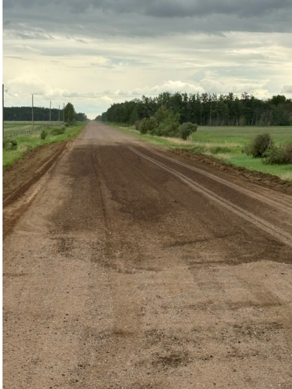
Public Works Figure 2.02. Road Patching Work with 1-1/2" Material
