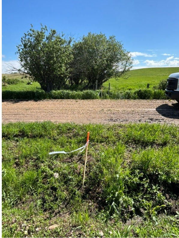
Public Works Figure 3.02. First Call Stakes for Culvert Install
