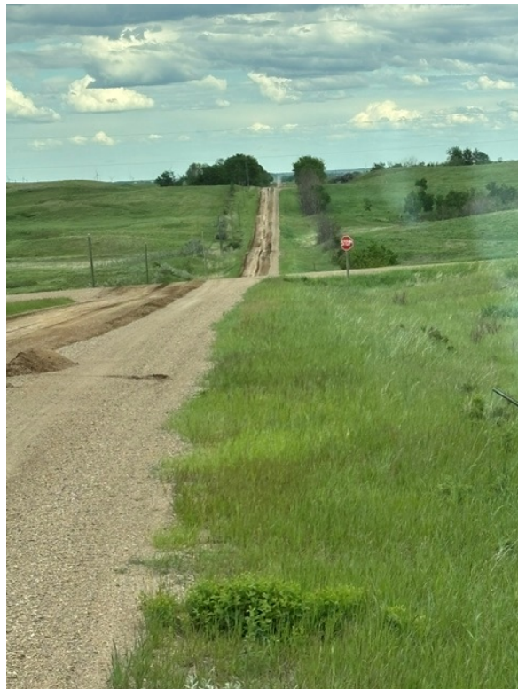
Public Works Figure 4.01. Blading Roads
