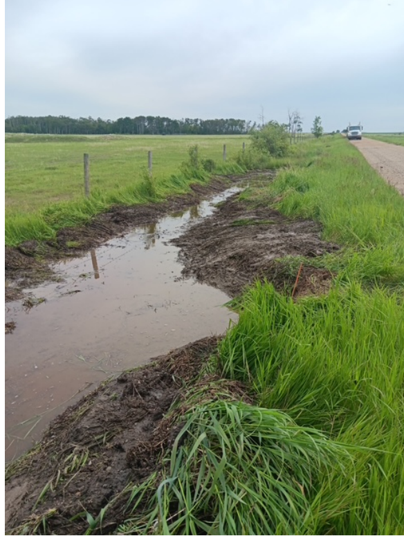
Public Works Figure 3.04. New Culvert Installation
