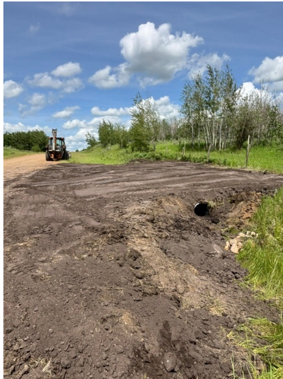
Public Works Figure 6.01. New Approach Install
