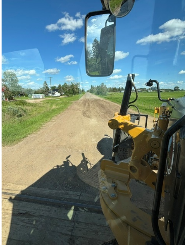
Public Works Figure 1.02. Road Patching Work
