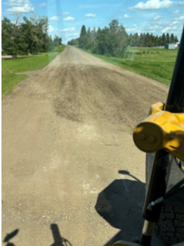
Public Works Figure 1.01. Road Patching Work
