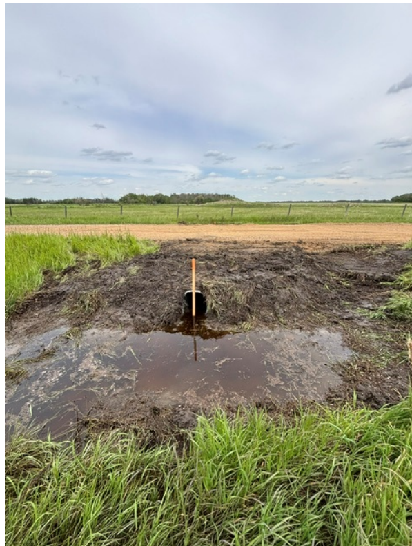
Public Works Figure 3.03. New Culvert Installation
