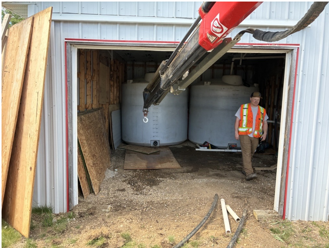
ASB Figure 6.01. Tank Install Walker Tankloader Station
