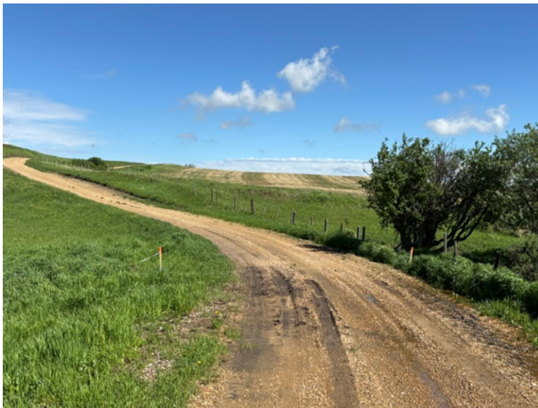
Public Works Figure 3.01. First Call Stakes for Culvert Install
