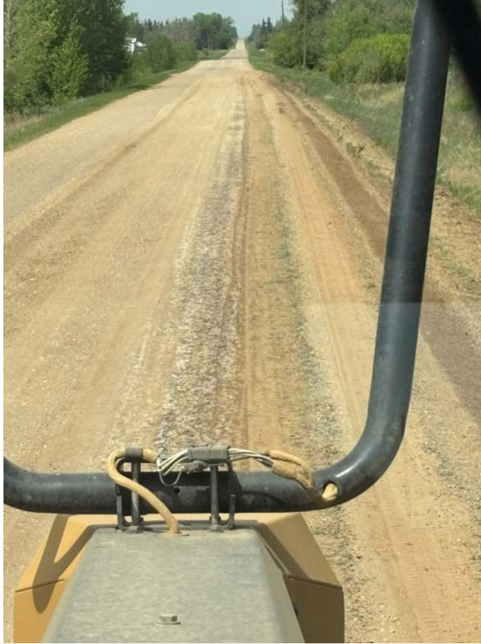
Public Works Figure 4.01. Road Shoulder Work with Grader
