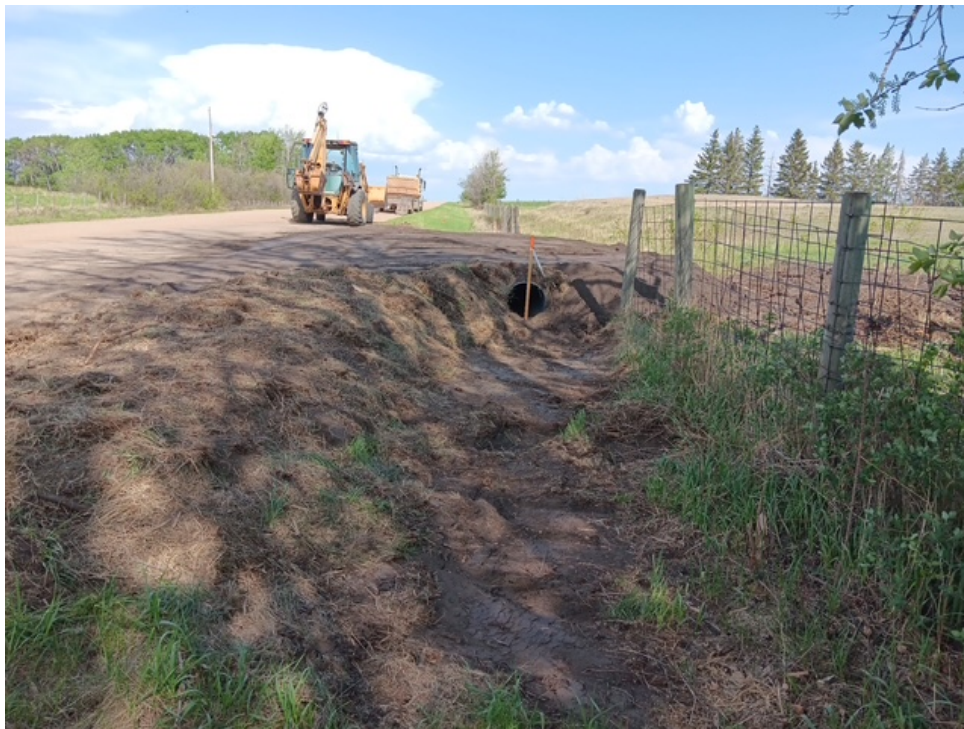
Public Works Figure 3.01. New Culvert Install
