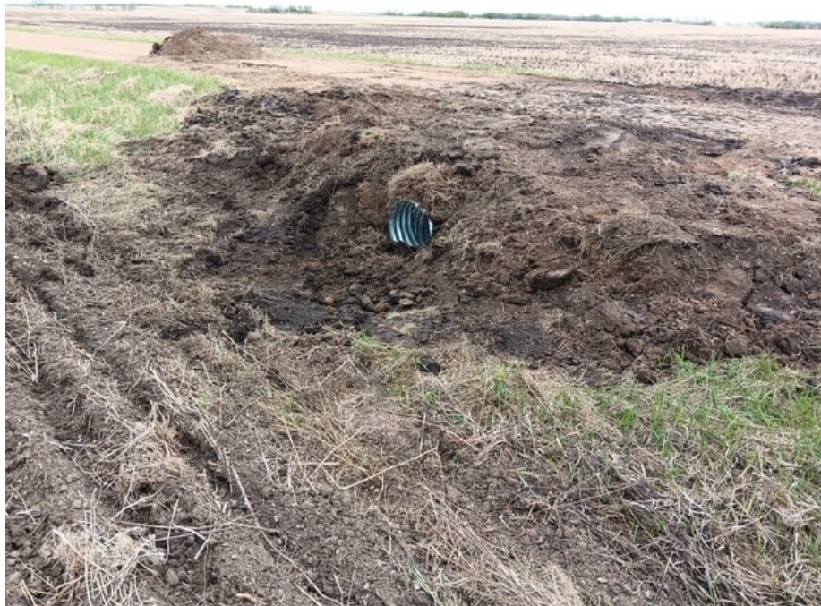
Public Works Figure 3.03. New Culvert Install
