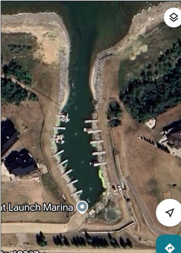
Projects, Engineering & Facilities Figure 1.02. Buffalo View Estates Aeration Motors Locations
