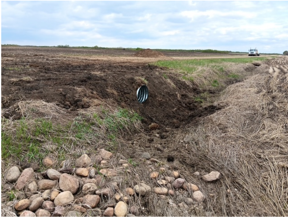
Public Works Figure 3.02. New Culvert Install
