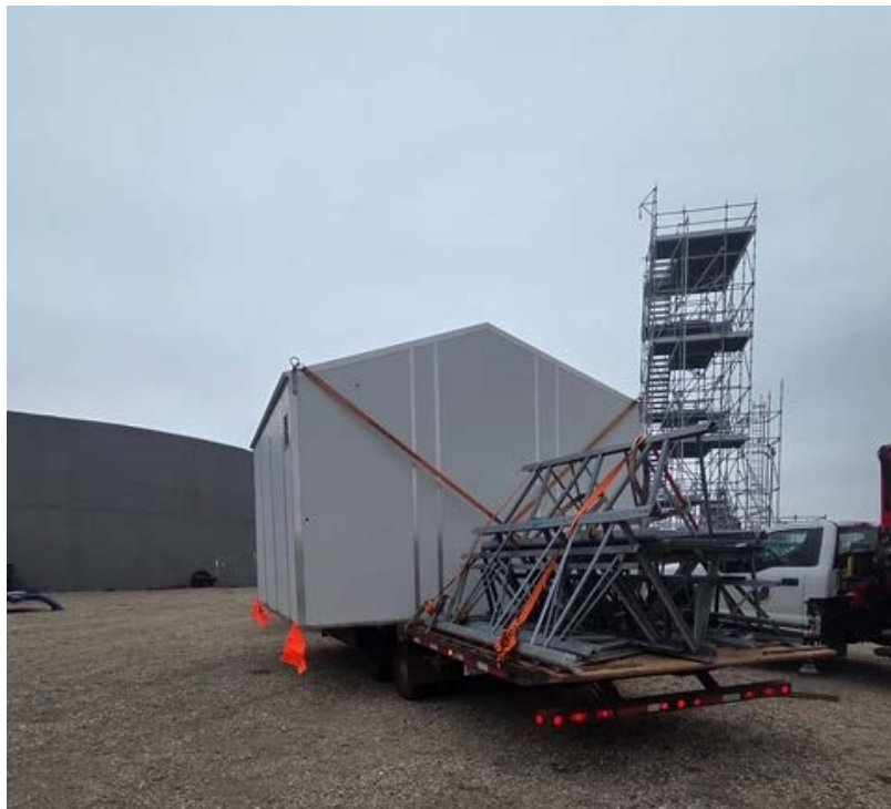
Public Works Figure 2.01. Shed Relocation
