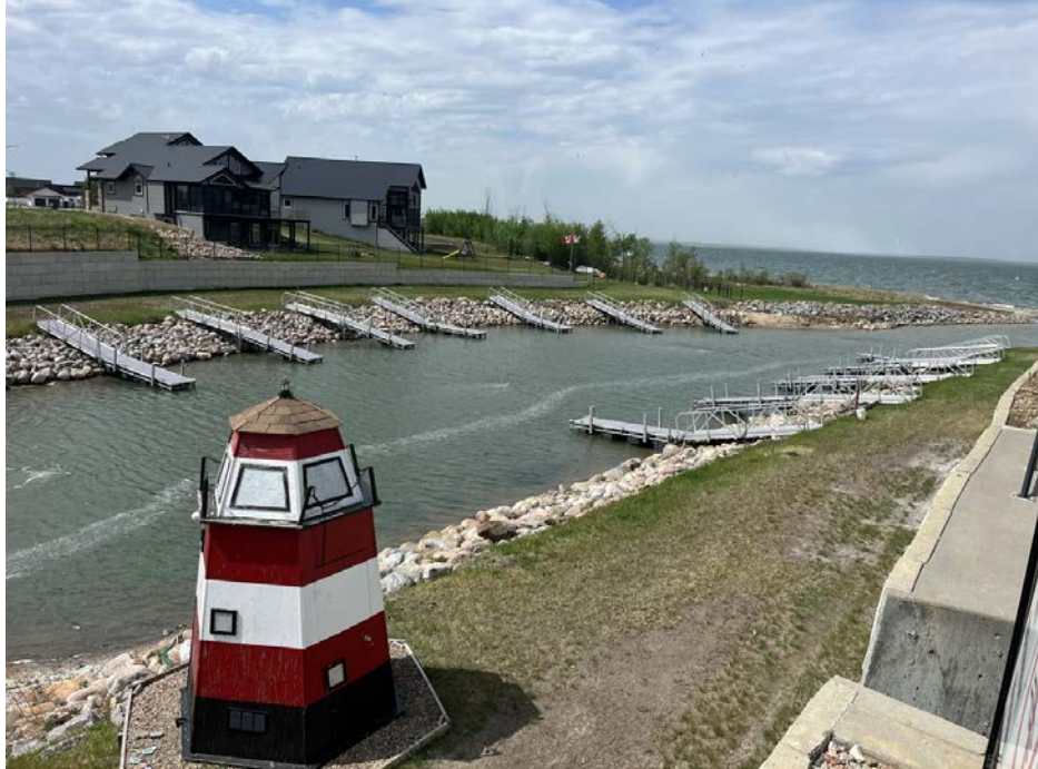
Projects, Engineering & Facilities Figure 1.03. Buffalo View Estates Marina Aeration Install
