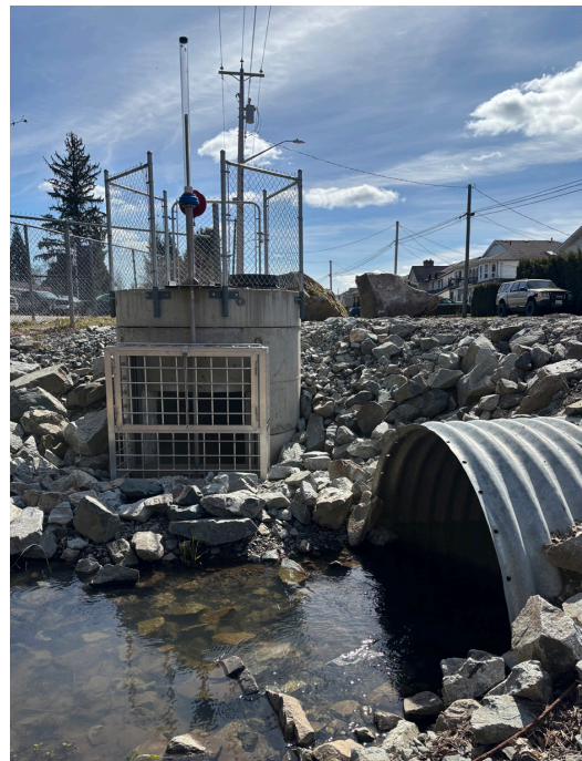
Above: Eby Storm Inlet Repair
