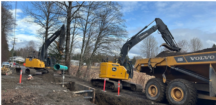
Above: Eby Street storm drain replacement
