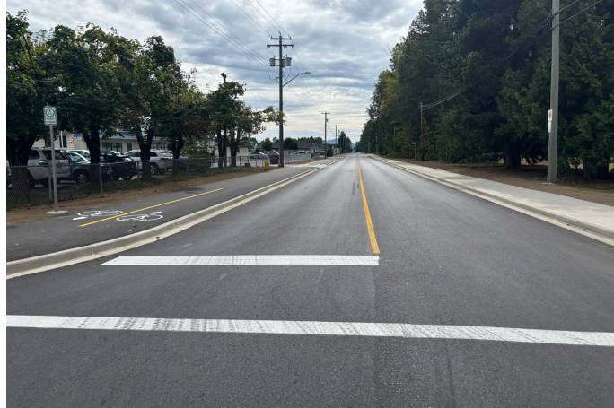
Above: Thomas Street Reconstruction Project
