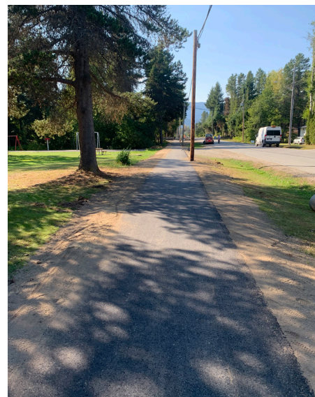
Above: Agar Avenue sidewalk replacement
